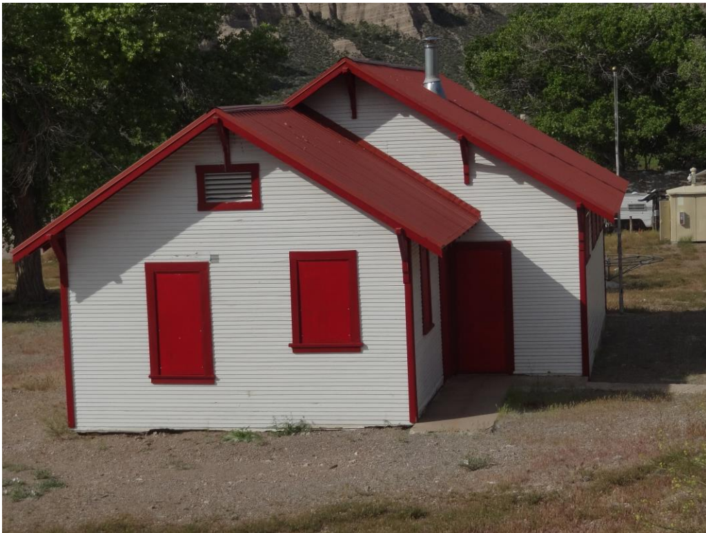
Elgin School House - Building #2537 Description: Rear addition in need of a concrete foundation.
