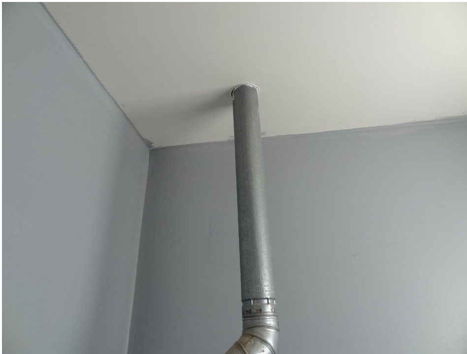
BDSP Park Residence - Building #0997 Description: Water Heater Flue Clearance to Combustible Project.
