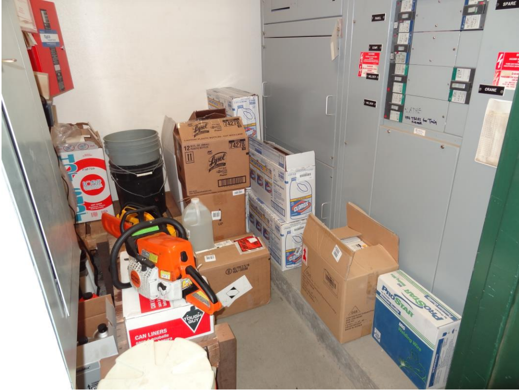
Boulder City Museum Maintenance - Building #0841 Description: Clearance at electrical panels needed.
