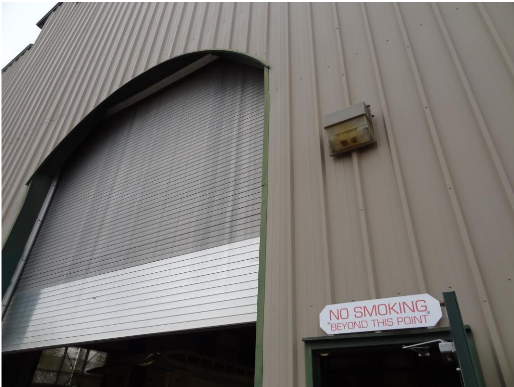
Boulder City Museum Maintenance - Building #0841 Description: Overhead door replacement needed.
