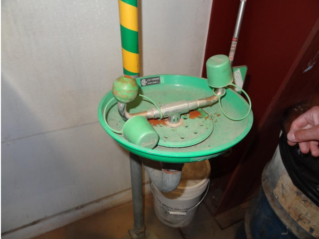
Boulder City Museum Maintenance - Building #0841 Description: Emergency eye wash station refurbishment needed.
