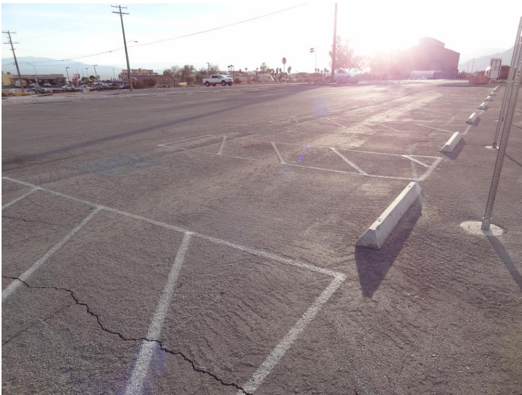
Boulder City Railroad Museum - Site #9951 Description: Slurry seal asphalt paving needed.
