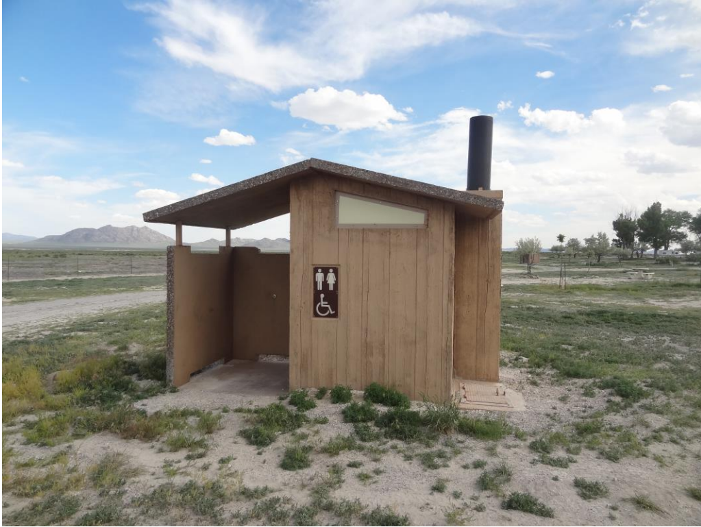
CXT Restroom #2 - Building #2326 Description: ADA accessible path of travel needed.
