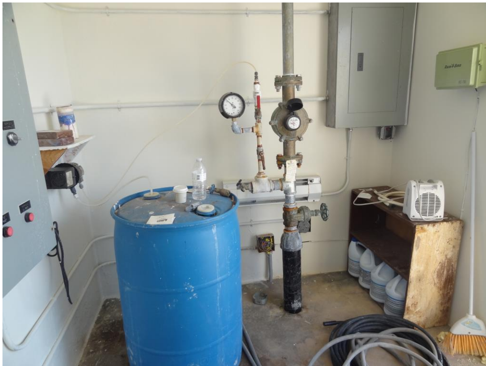
Kirch WMA Pump House - Building #0644 Description: Clearance needed at electrical panel.
