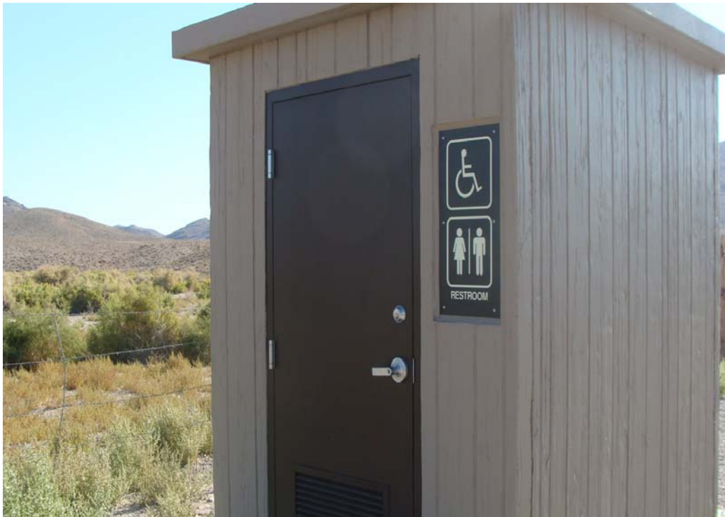
CXT Comfort Station #1 - South - Building #2942 Description: Exterior of the structure.
