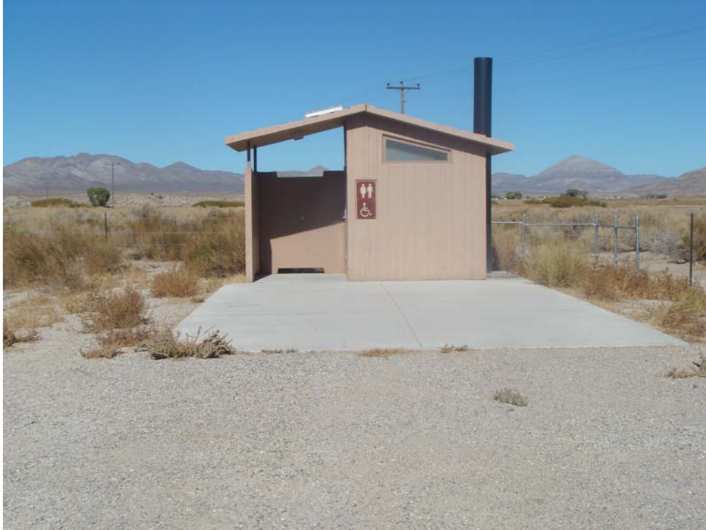
CXT Comfort Station #2 - North - Building #3028 Description: Exterior of the structure.
