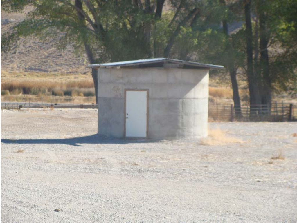
Granary - Building #0904 Description: Exterior of the structure.
