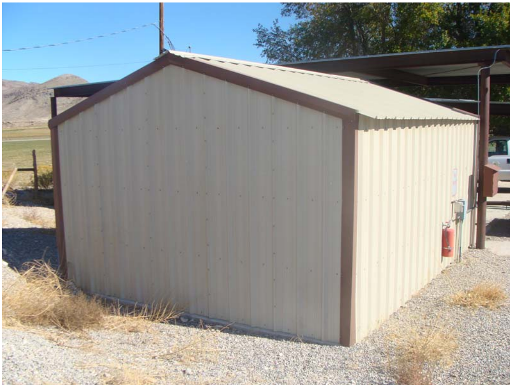
WMA Storage Building - Building #3029 Description: Exterior of the structure.
