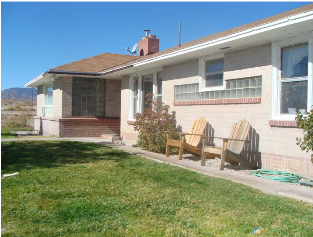
WMA Supervisor's Residence - Building #0903 Description: Exterior of the structure.
