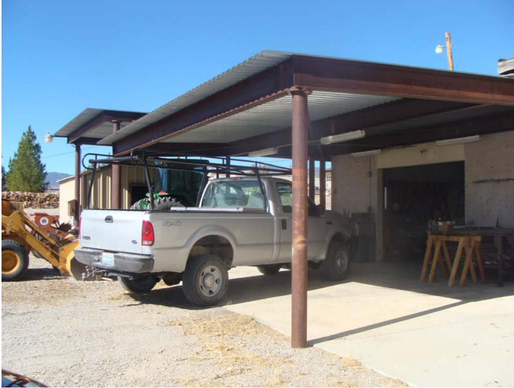
Maintenance Shop - Building #0647 Description: Exterior of the building.
