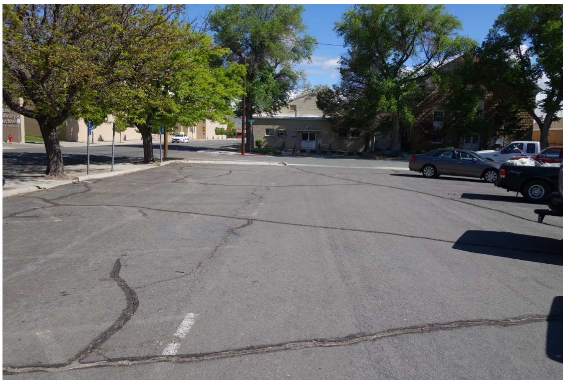
B & G Office Site - Site #9956 Description: South Parking Lot Crack Fill & Seal.
