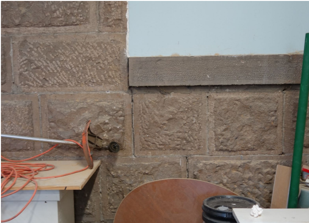
B & G Office - Building #0391 Description: Cracks in the Unreinforced Wall Structure.
