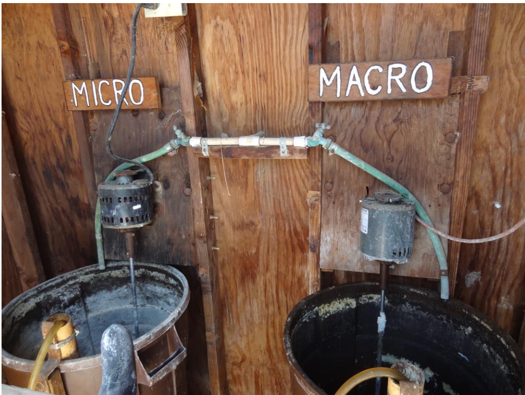
Nursery Fertilization Shed - Building #3045 Description: Fertilizer injector replacement needed.
