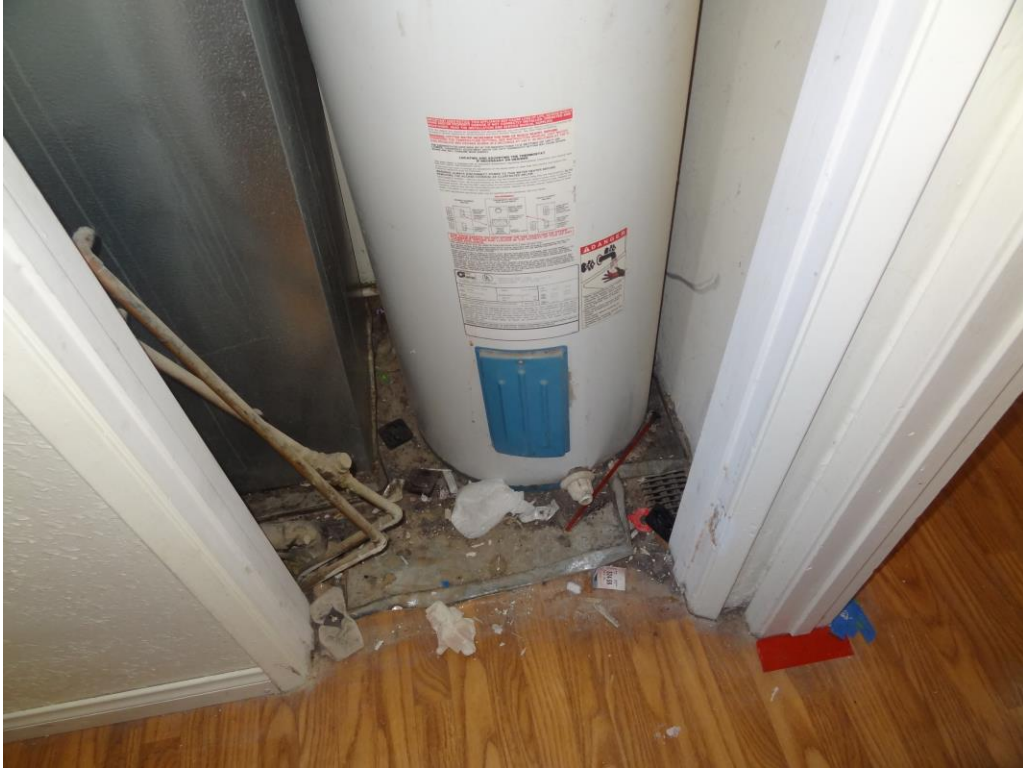
Nursery Residence - Building #3046 Description: Damaged subfloor needs to be replaced.
