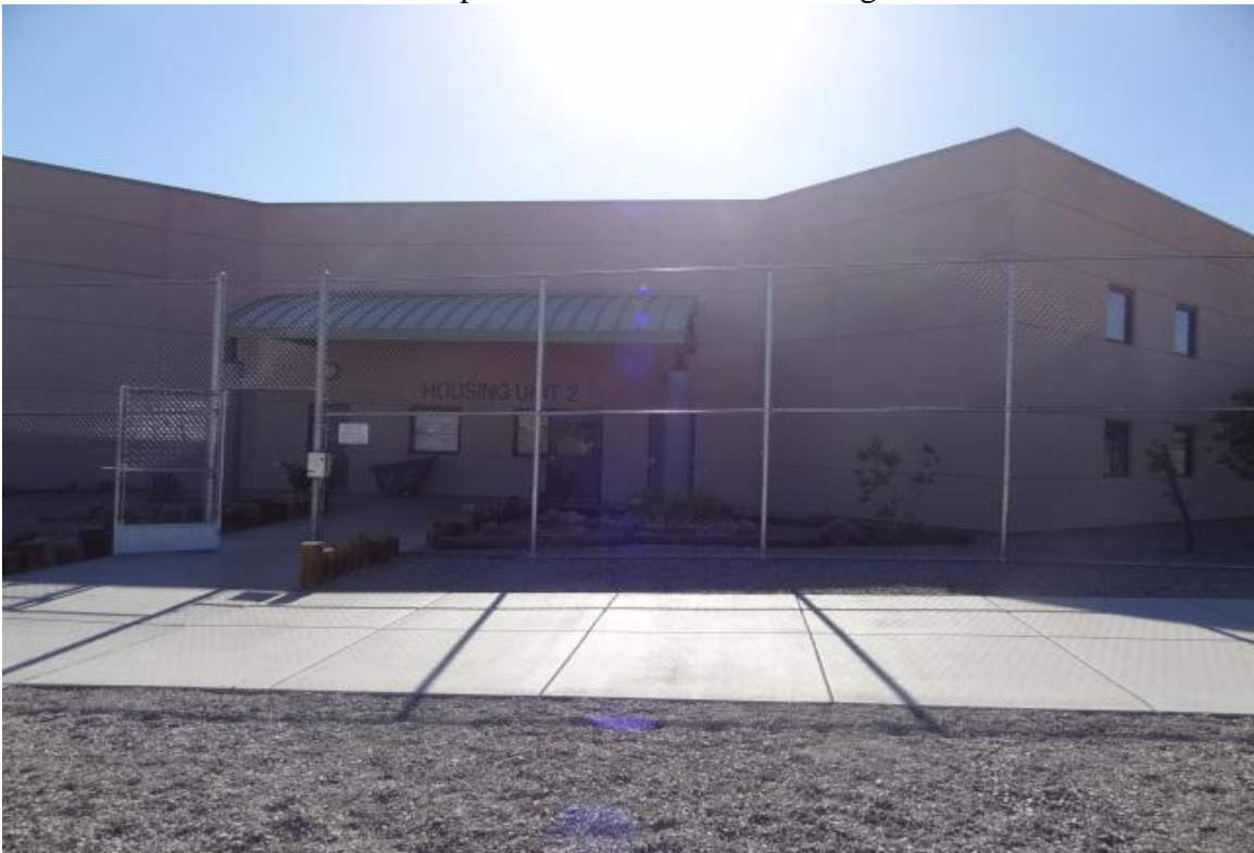
Housing Unit A2 – FCA Building #3089 Description: Exterior of the building.
