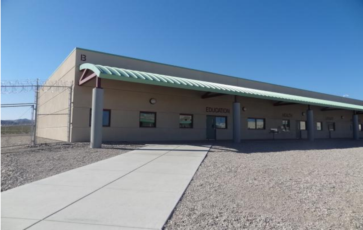
Inmate Services B – FCA Building #3090 Description: Exterior of the building.
