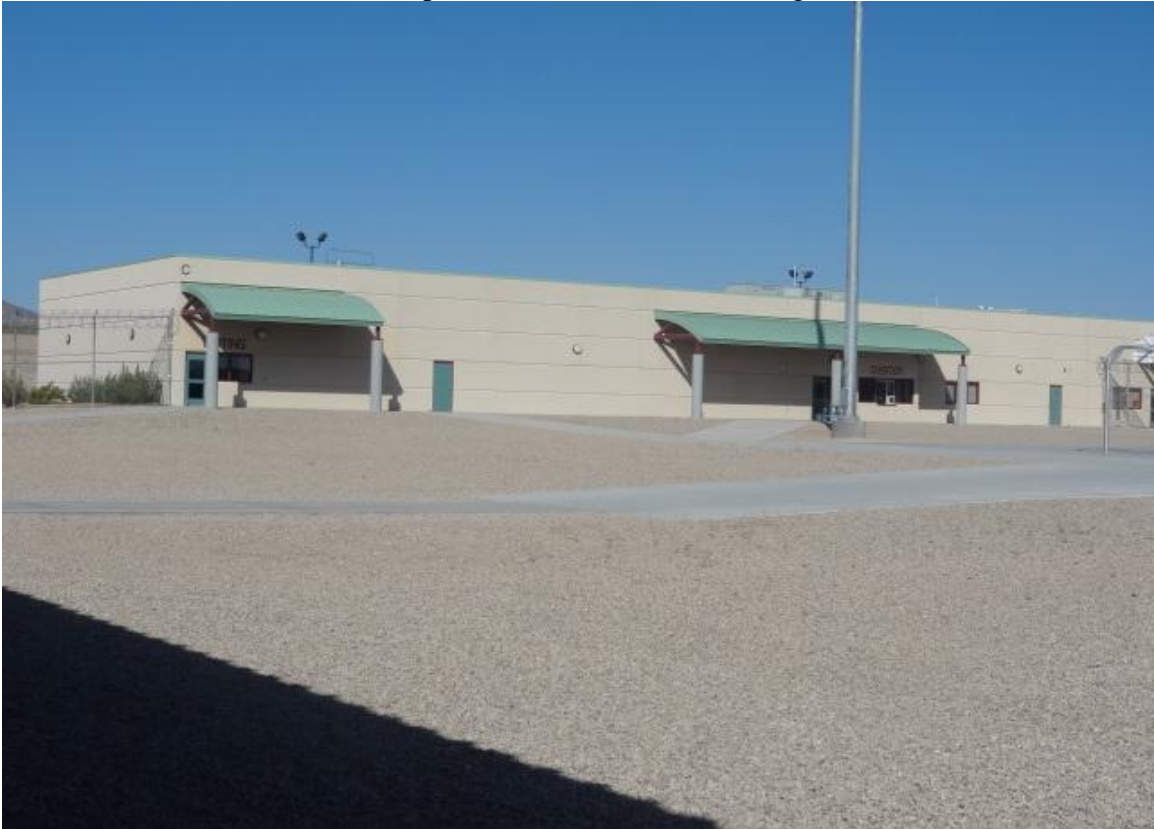
NDOC / NDF Administration C – FCA Building #3091 Description: Exterior of the building.
