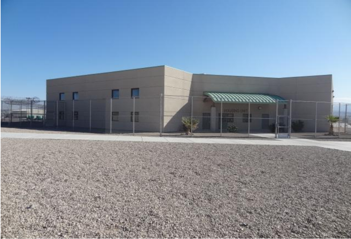
Housing Unit A1 – FCA Building #3088 Description: Exterior of the building.
