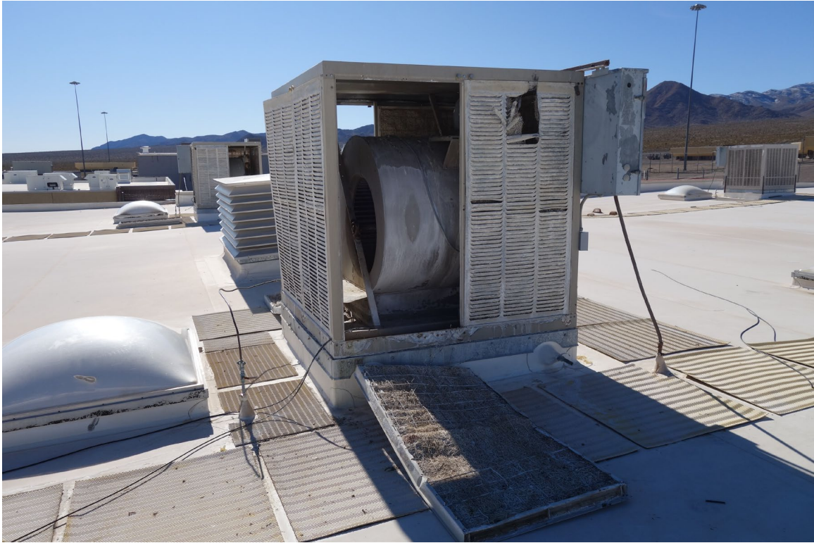
SDCC Industrial/Culinary/ P.I. – FCA Building #0165 Description: Evaporative cooler in need of replacement.
