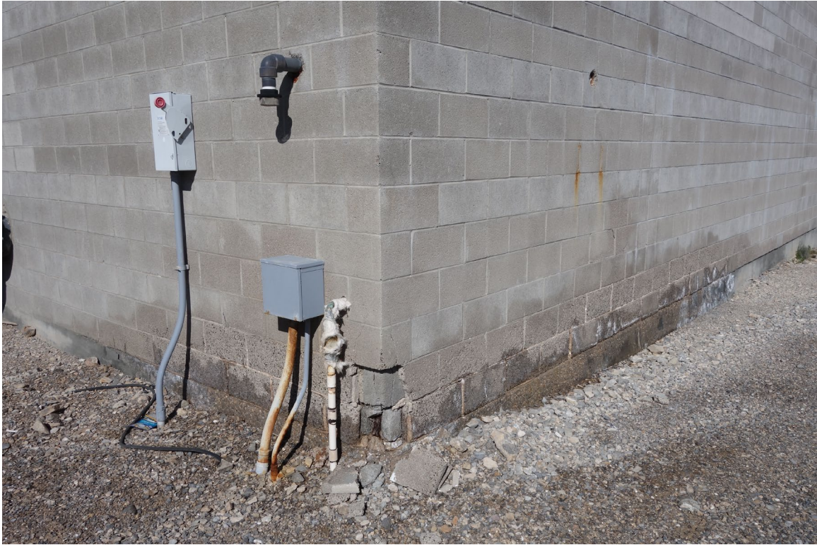
SDCC Pump House 1 (formerly Pump House 2) – FCA Building #2706 Description: Water damage from interior drainage problem.
