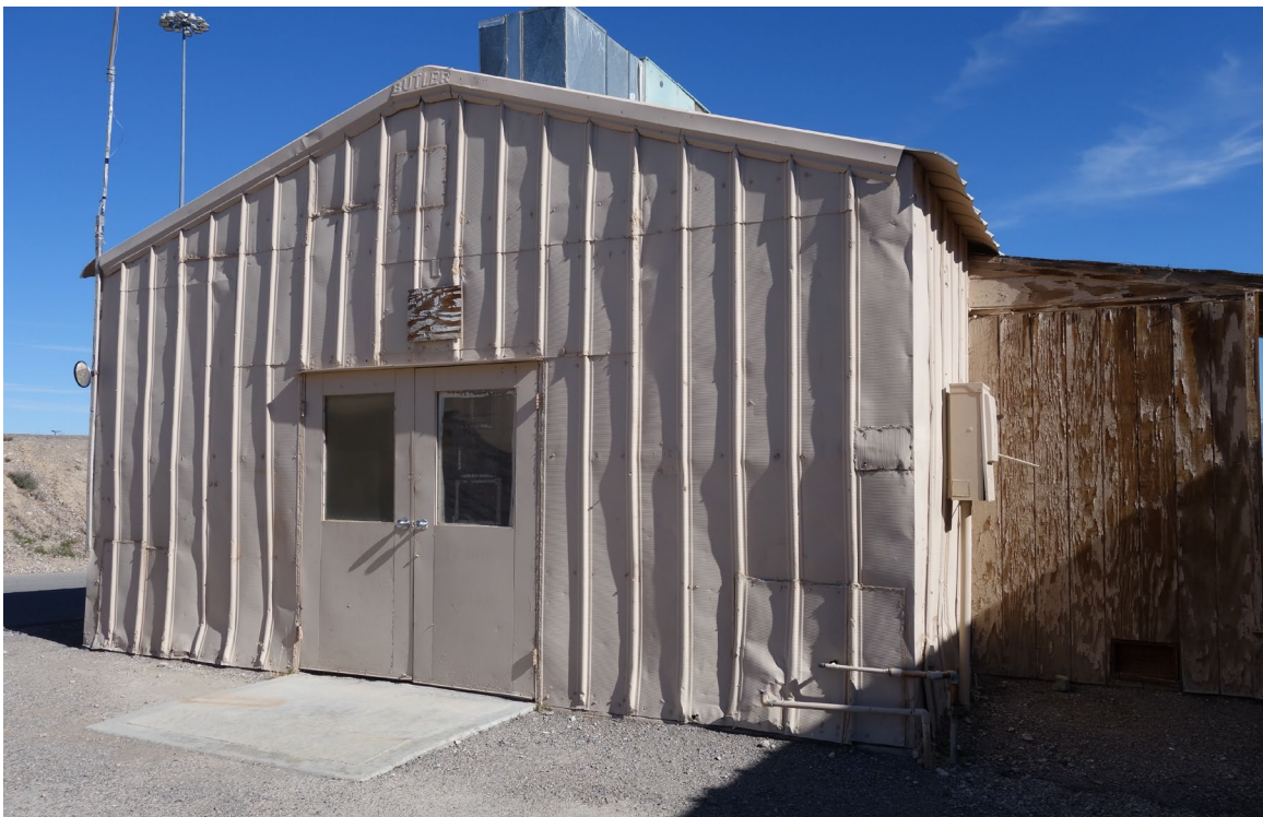
SDCC Upholstery Building (formerly Glass Shop) – FCA Building #2183 Description: Exterior siding in need of replacement.
