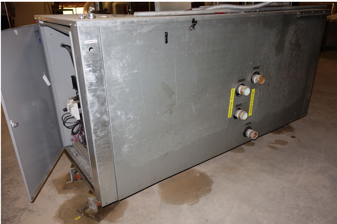
SDCC Housing Unit 6 – FCA Building #0162 Description: Failed domestic water heating unit (Templifier).
