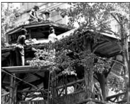
Central Park has developed an in-house historic preservation crew to undertake small projects. A specialized crew has been trained to repair and rebuild rustic furnishings. Photo: Central Park Conservancy.
