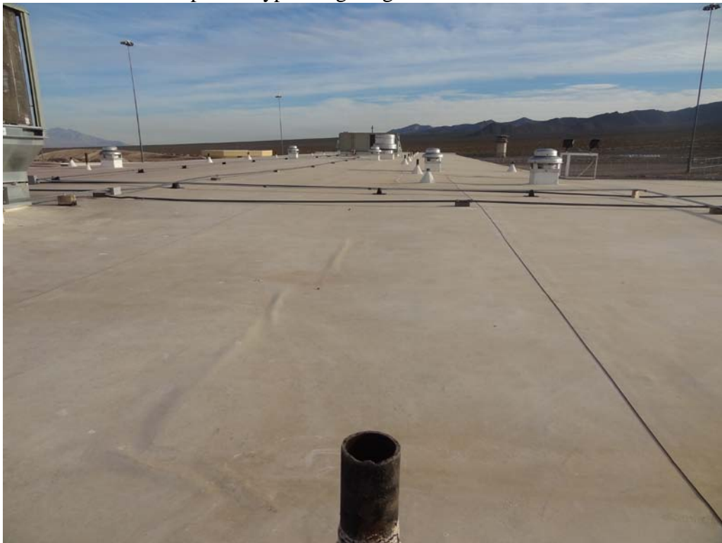
Housing Unit #8 – FCA Building #1481 Description: 14 year old single-ply roof membrane.
