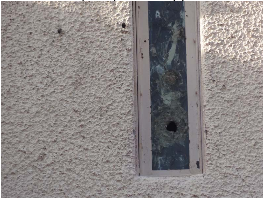
Housing Unit #8 – FCA Building #1481 Description: Typical cell window.
