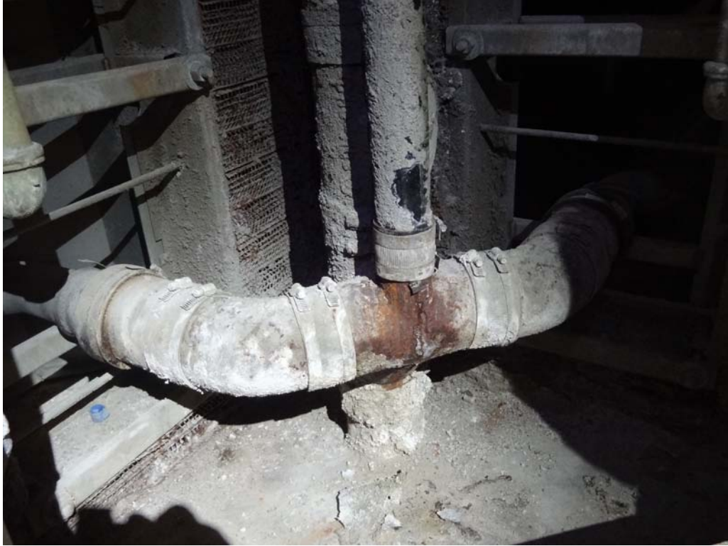
Housing Unit #8 – FCA Building #1481 Description: Typical plumbing chase between cells.
