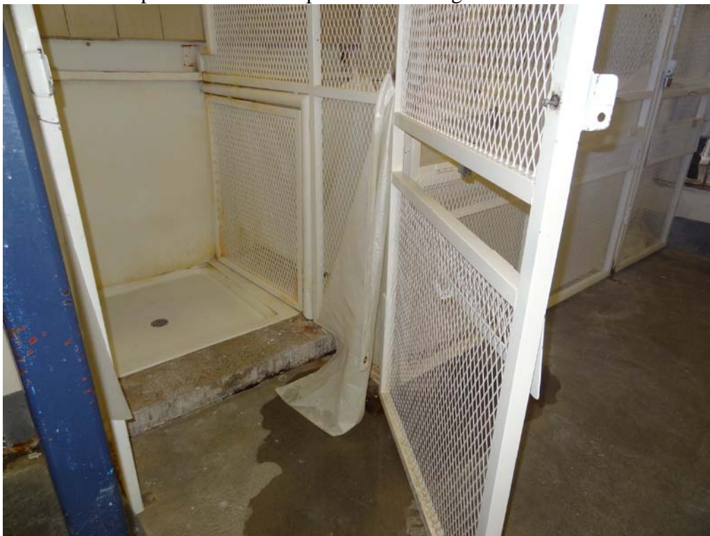
Housing Unit #8 – FCA Building #1481 Description: Typical shower enclosure.
