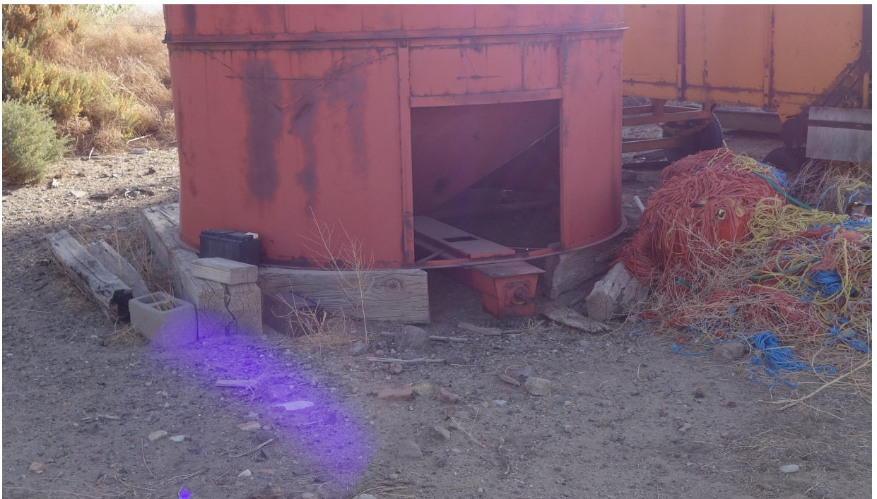
Silo 2 – FCA Building #3868 Description: Silo 2 on Unstable Wood Foundation.
