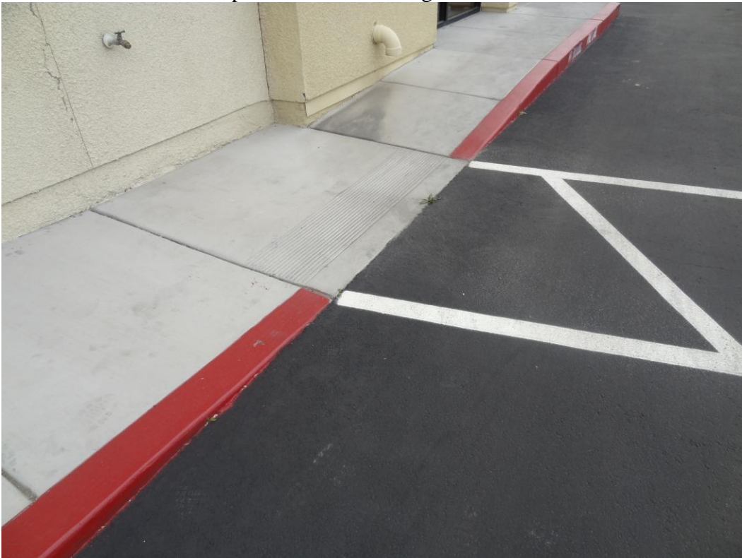
Fleet Services – Las Vegas – FCA Building #3155 Description: ADA Path of Travel
