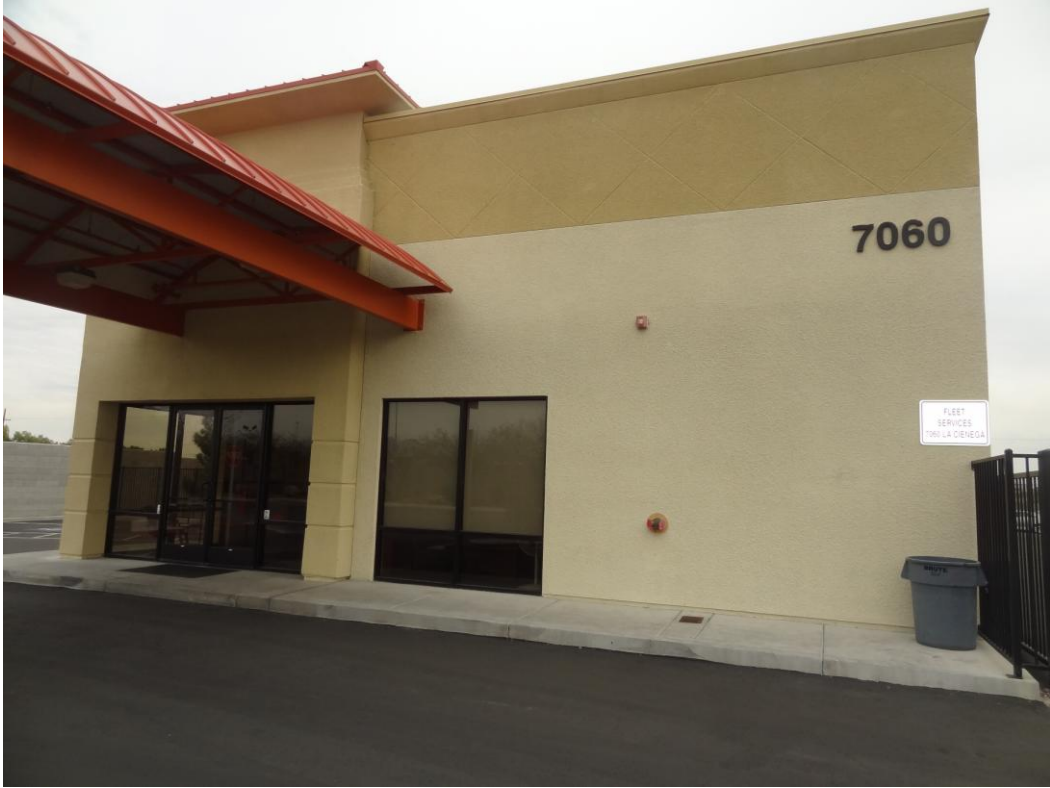
Fleet Services – Las Vegas – FCA Building #3155 Description: Entrance facing Bonanza Blvd.
