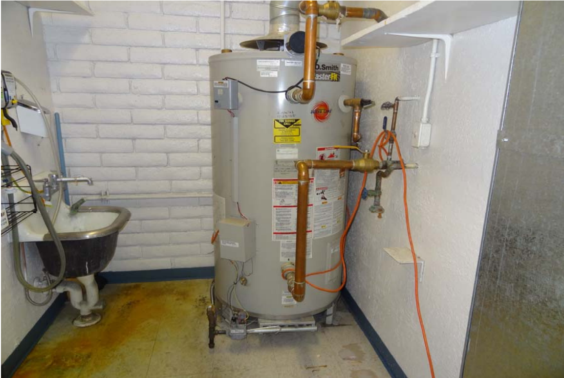
Old Las Vegas Metro Police Station - Building #3113 Description: View of the water heater.
