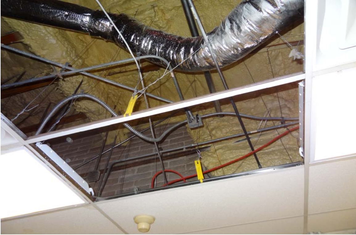
Old Las Vegas Metro Police Station - Building #3113 Description: Missing ceiling tiles.
