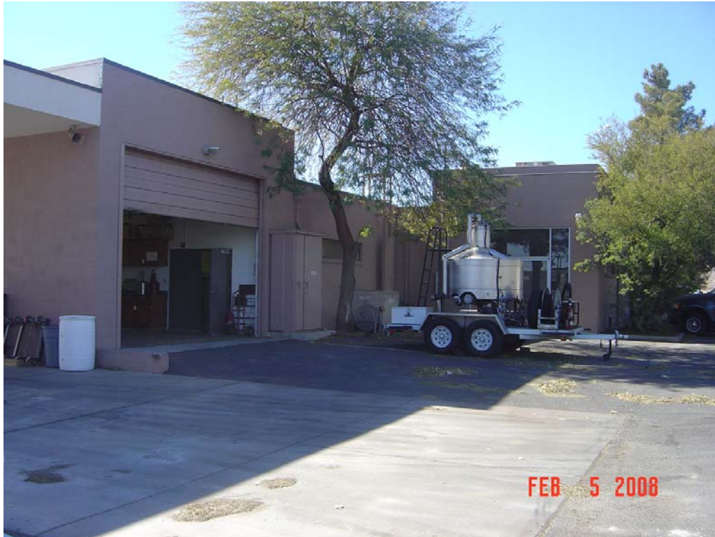
Agriculture Office - Building #0418 Description: Exterior of the building.
