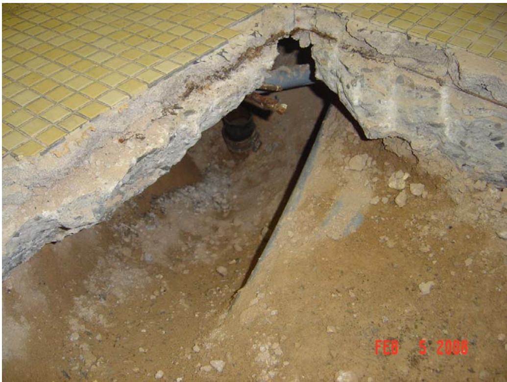
Agriculture Office - Building #0418 Description: Restroom drain repair.
