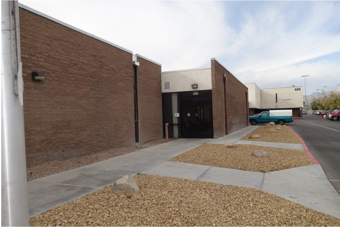
Belrose Office Building - Building #0286 Description: Exterior Wall Pack Lighting Upgrade Recommended.
