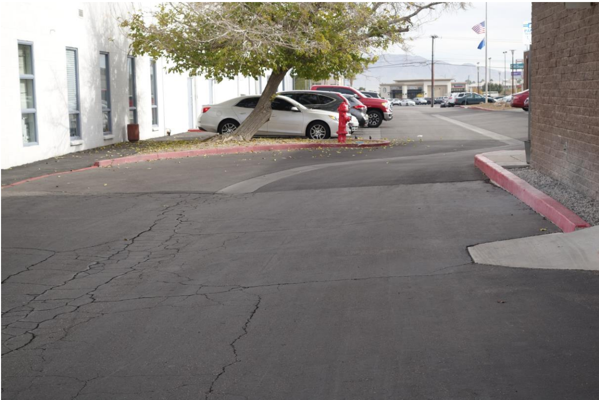
Belrose Office Building Site - Site #9831 Description: Slurry Seal Paving in East Parking Area.
