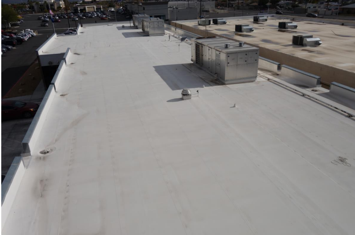
Belrose Office Building - Building #0286 Description: Guard Installations at Unprotected Edges Near Equipment.
