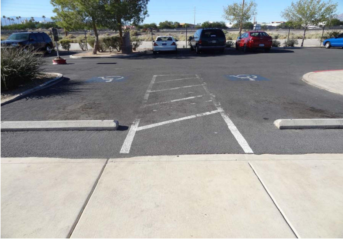
DMV Express Office Site - Site #9832 Description: View of ADA accessible parking.
