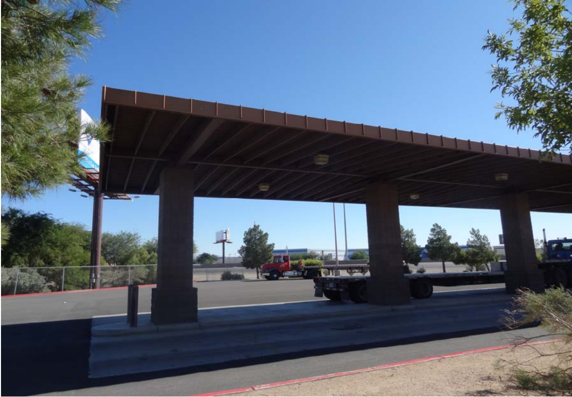
Inspection Station Canopy - Building #3106 Description: Exterior of the structure.
