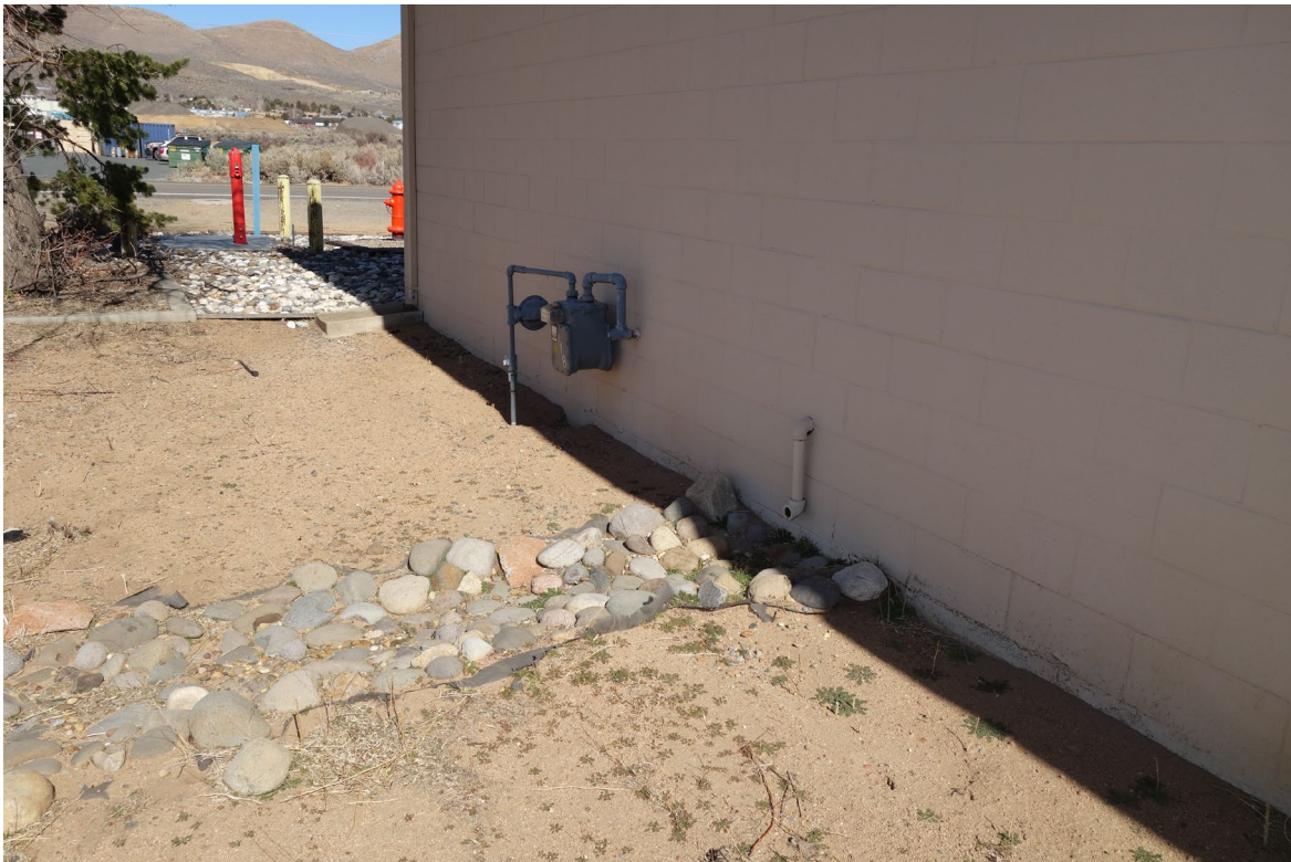
Marjorie Russell Research Center – FCA Building #0208 Description: Seismic Gas Isolation Valve Needed.
