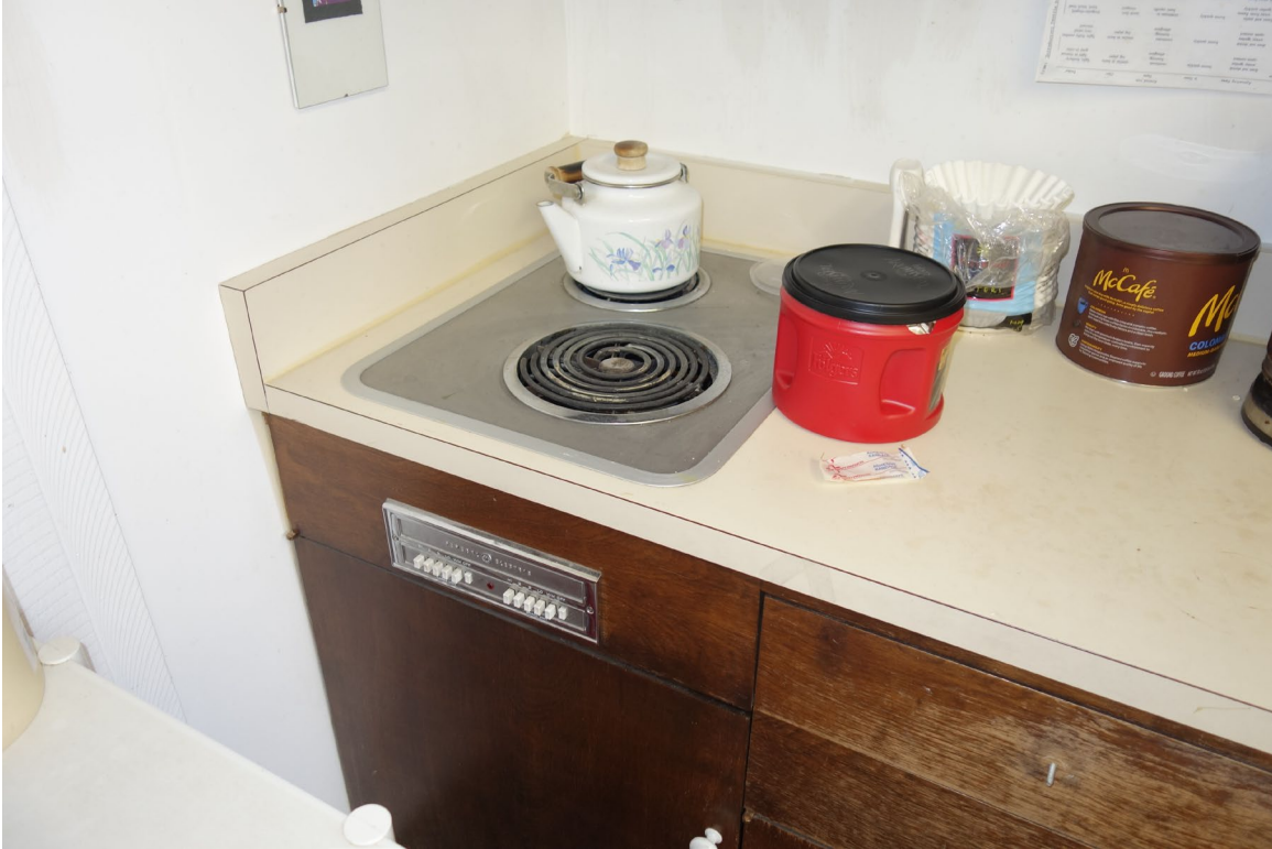
Marjorie Russell Research Center – FCA Building #0208 Description: Breakroom Remodel and Exhaust Ventilation Recommended.
