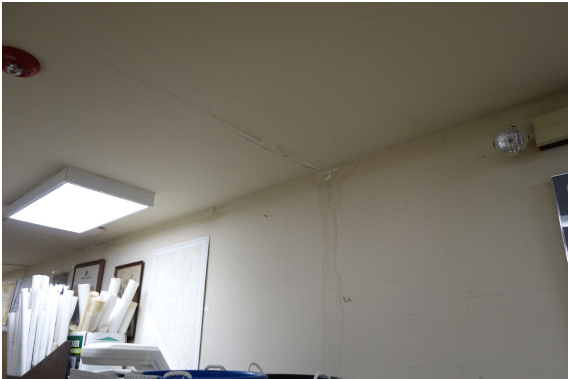
Nevada Historical Society - Building #0401 Description: Gypsum Board Repairs Needed.
