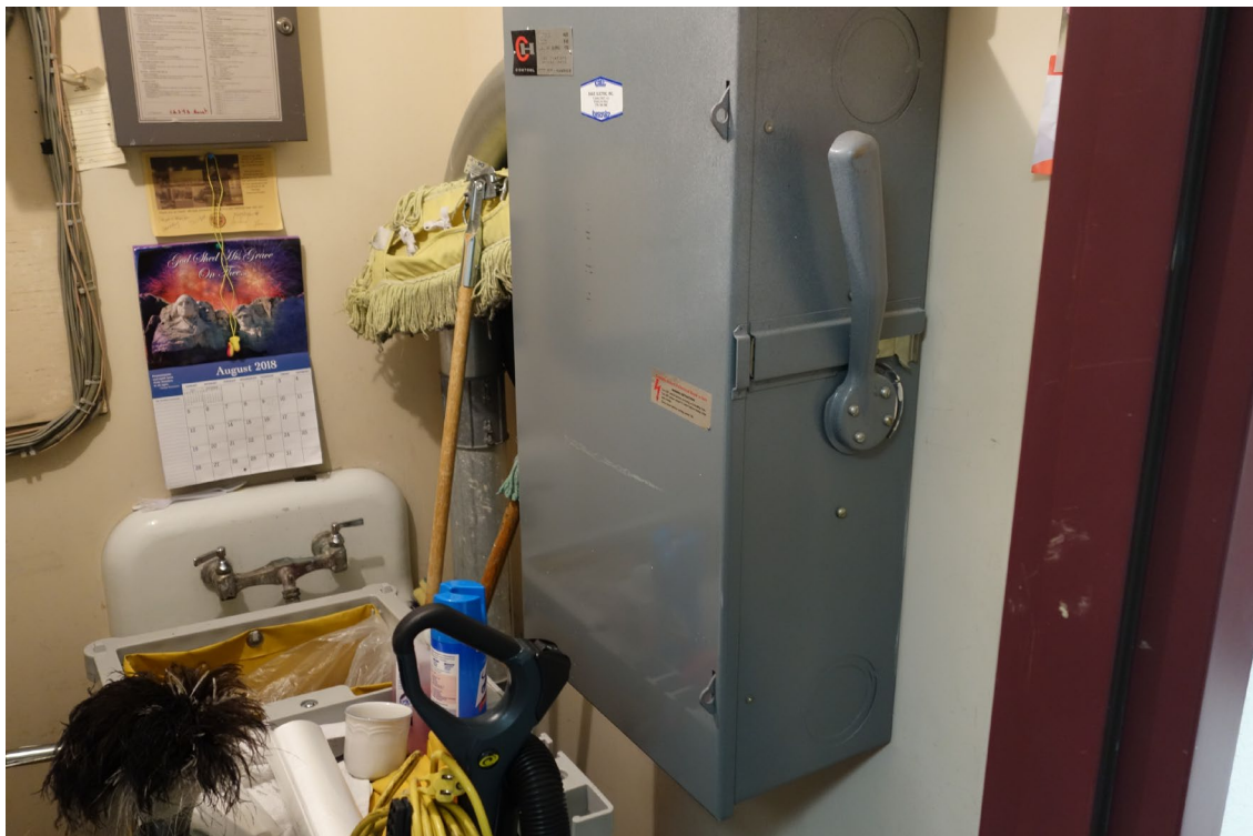
Nevada Historical Society - Building #0401 Description: Clearance at Electrical Equipment Required.
