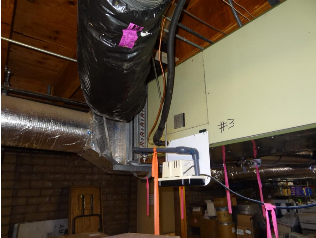
Nevada Early Intervention Services - Building #0515 Description: HVAC Replacement.
