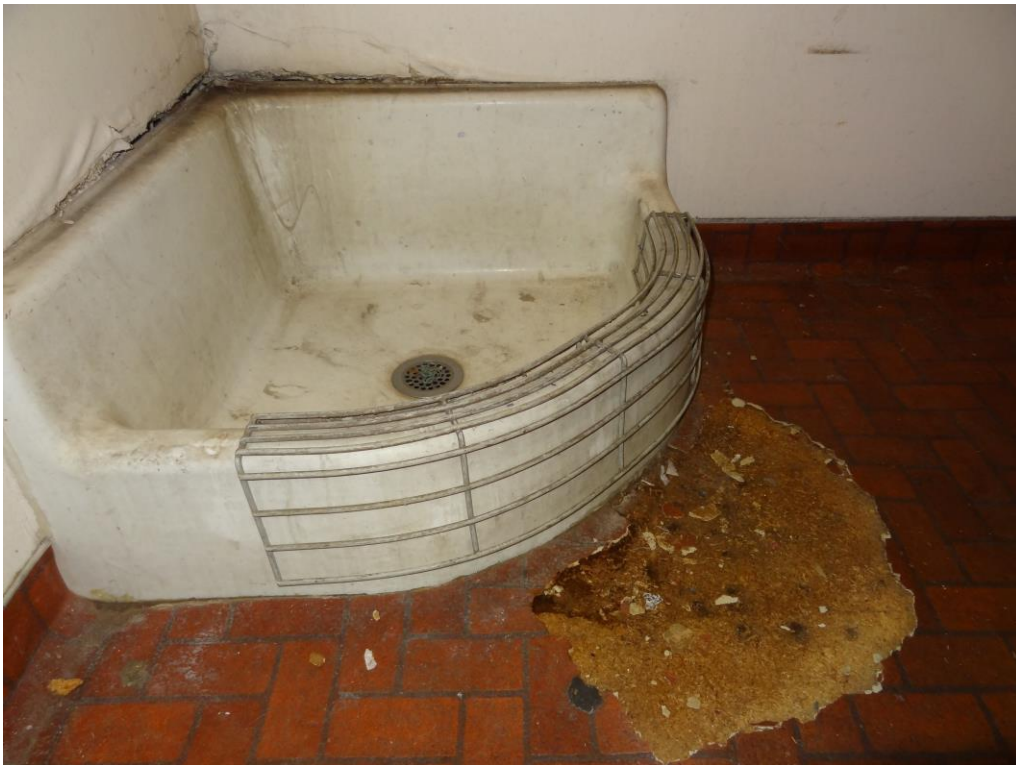
Nevada Early Intervention Services - Building #0515 Description: Janitors Closet Repairs.
