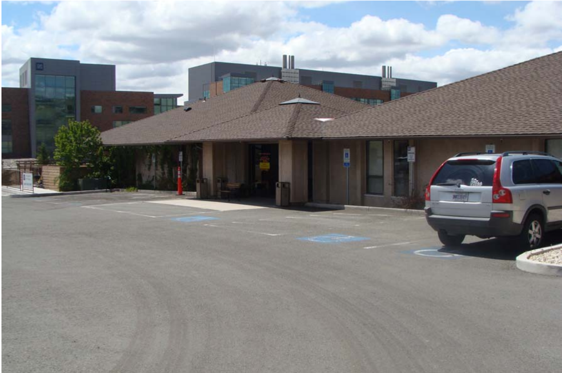
Nevada Early Intervention Services Site - Site #9859 Description: ADA accessible parking at building entrance.
