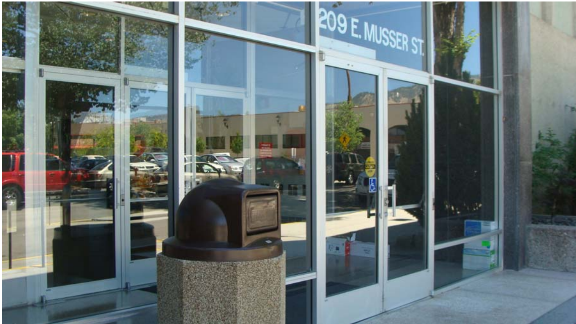
Blasdel Office Building Site - Site #9860 Description: ADA accessible entrance.
