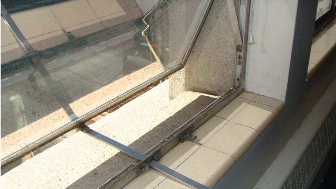
Blasdel Office Building - Building #0200 Description: Typical operable window installation.
