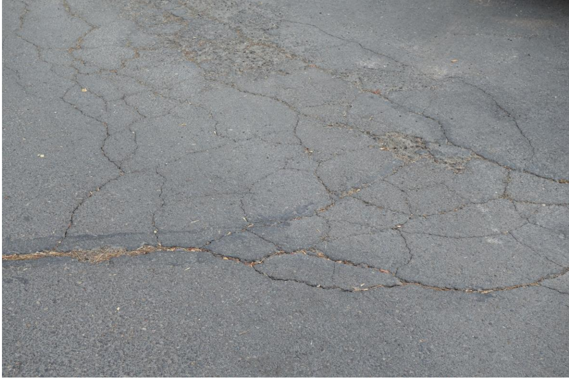
Carson City Motor Pool Site - Site #9862 Description: Failing Parking Pavement.
