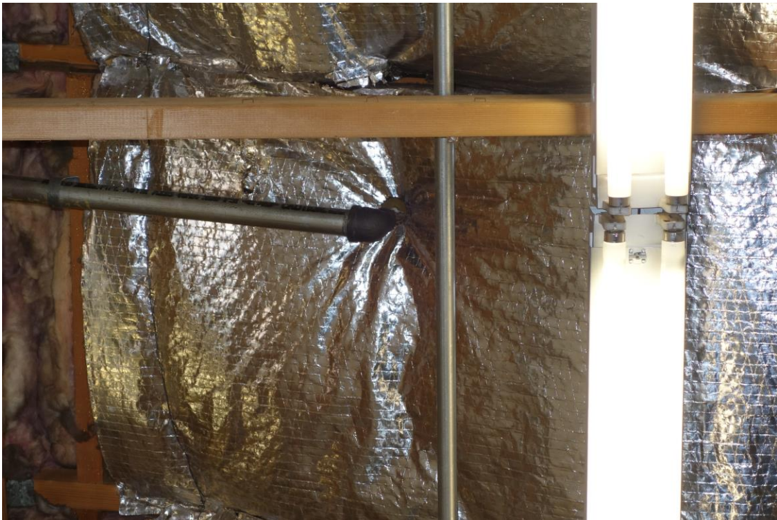
Carson City Motor Pool - Building #0204 Description: Insulation Repairs and Fire Sprinkler Clearance.
