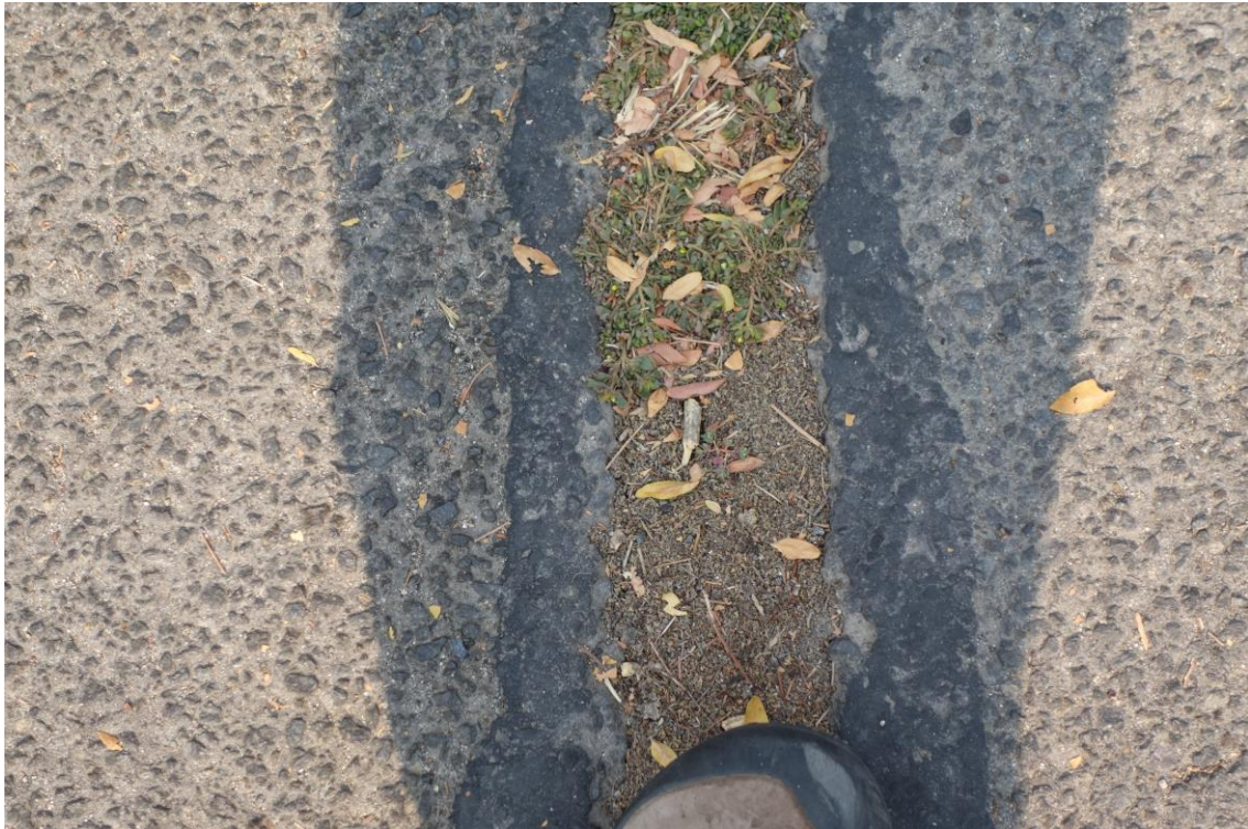
Carson City Motor Pool Site - Site #9862 Description: Parking Pavement Patch, Crack, and Surry Seal.
