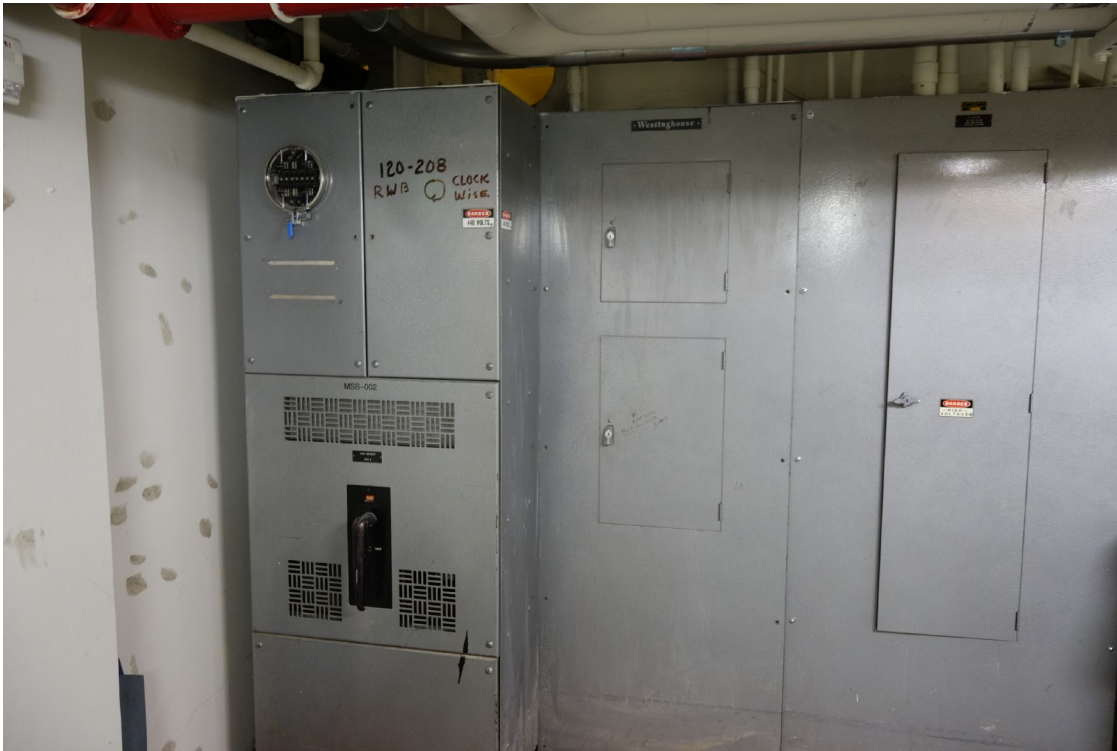
Carson City State Offices Building - Building #0397 Description: Electrical Arc Flash & Coordination Study Needed.
