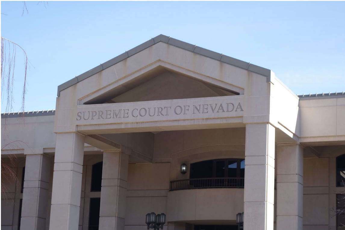
Supreme Court of Nevada - Building #1478 Description: View of Exterior Metal Finishes.
