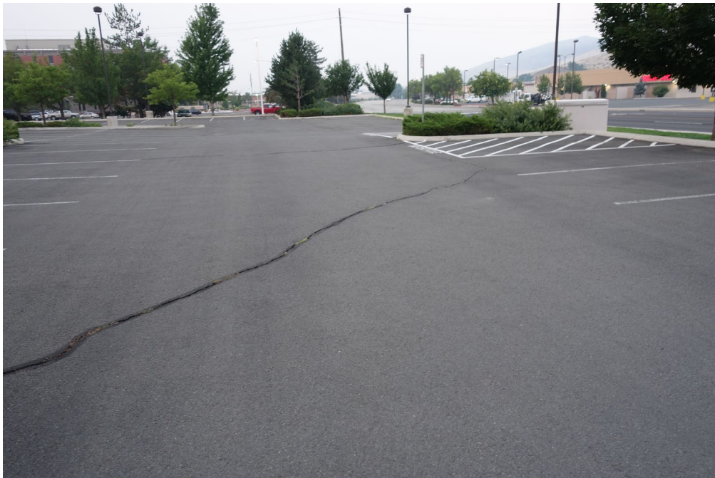
Richard H. Bryan Building - Site #9867 Description: Crack Fill & Seal Needed.
