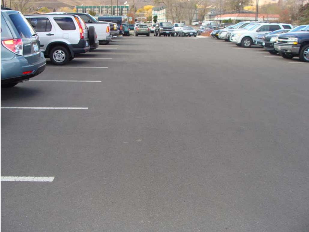
Richard H. Bryan Building - Site #9867 Description: Parking lot on north side.
