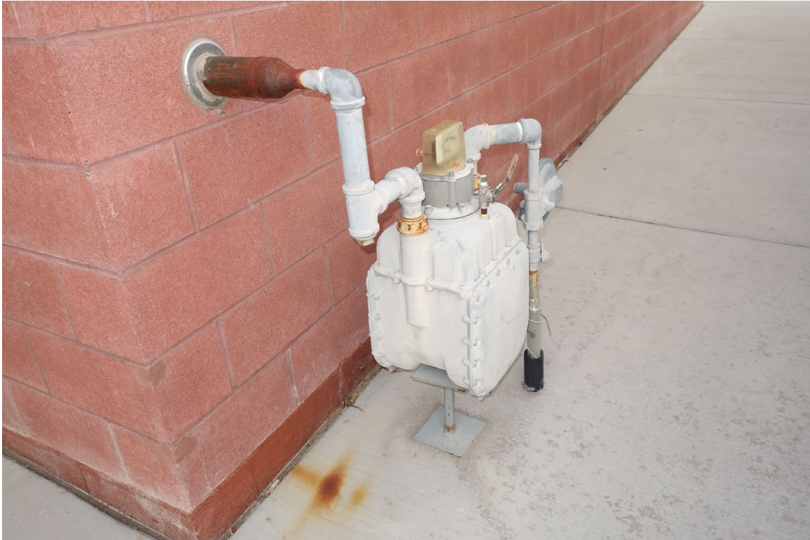
North Decatur DMV Services Center - Building #2453 Description: Seismic Gas Shut-Off Valve Needed.
