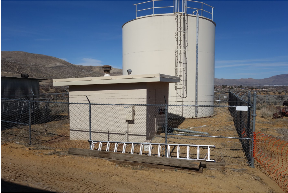
Indian Hills Pump House – FCA Building #0859 Description: Exterior of the Building.
