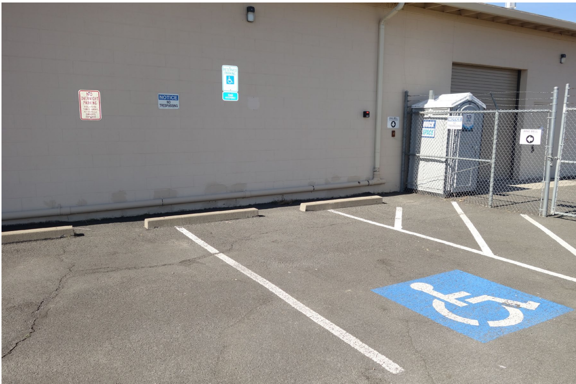
Nevada State Museum Indian Hills Site – FCA Site #9874 Description: ADA Accessible Parking Space.
