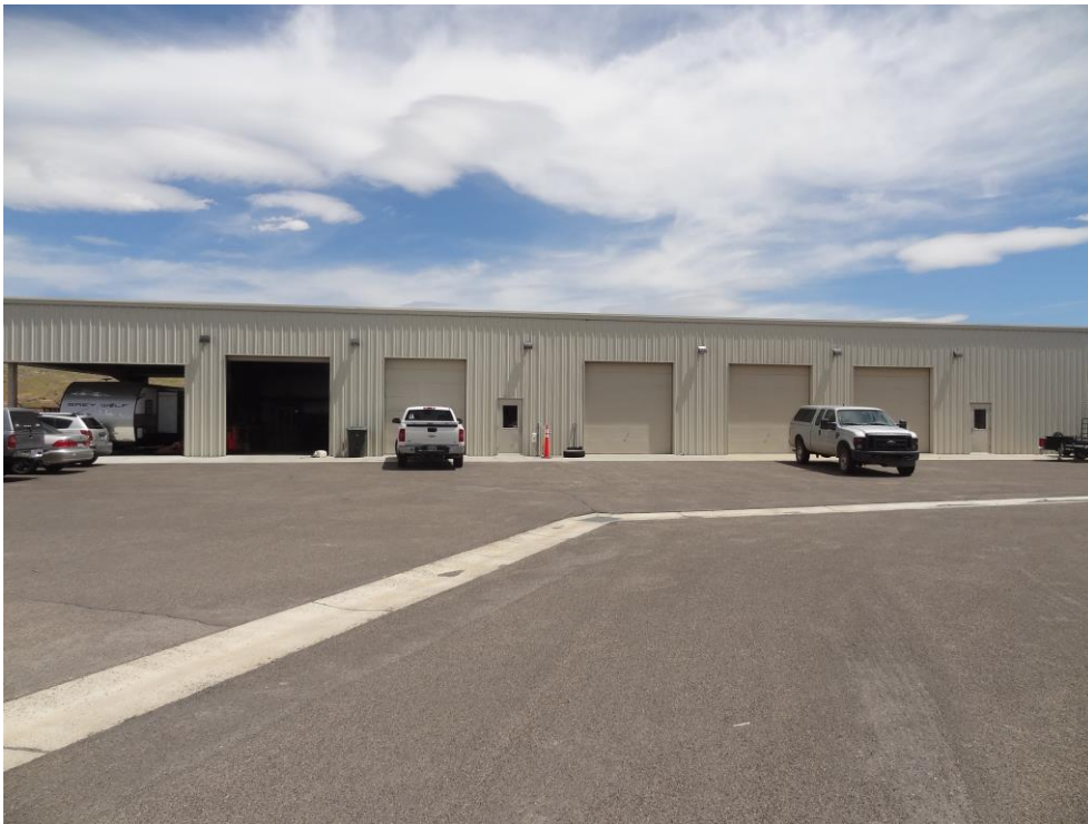
Elko Eastern Region Garage - Building #2298 Description: Exterior finishes needed.
