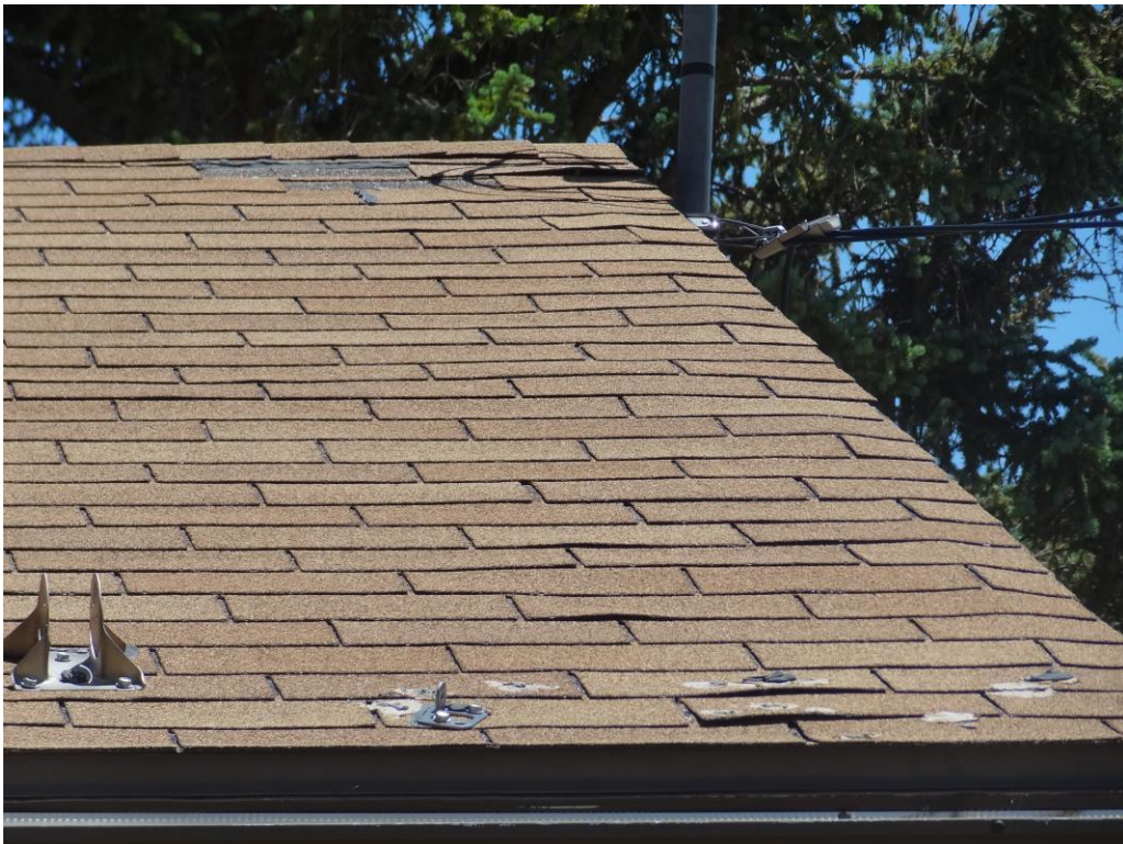
S.C. Rearing Station Residence #2 South - Building #0947 Description: Roof replacement needed.
