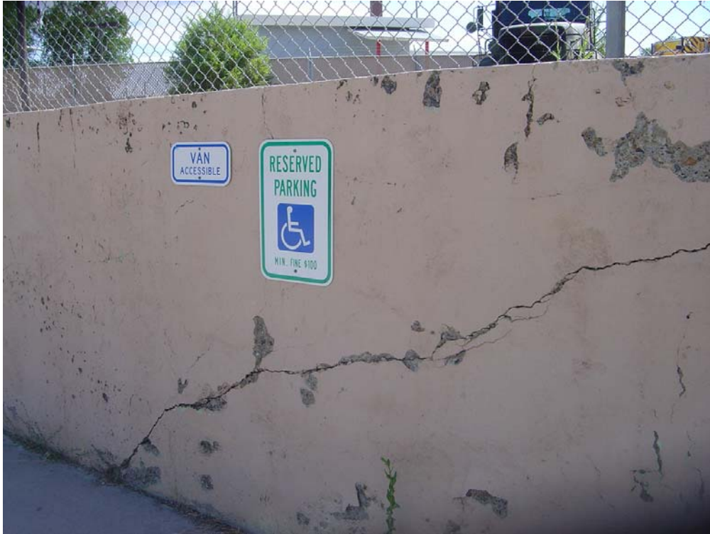
Nevada National Guard Site # 9884 Description: Damaged retaining wall.
