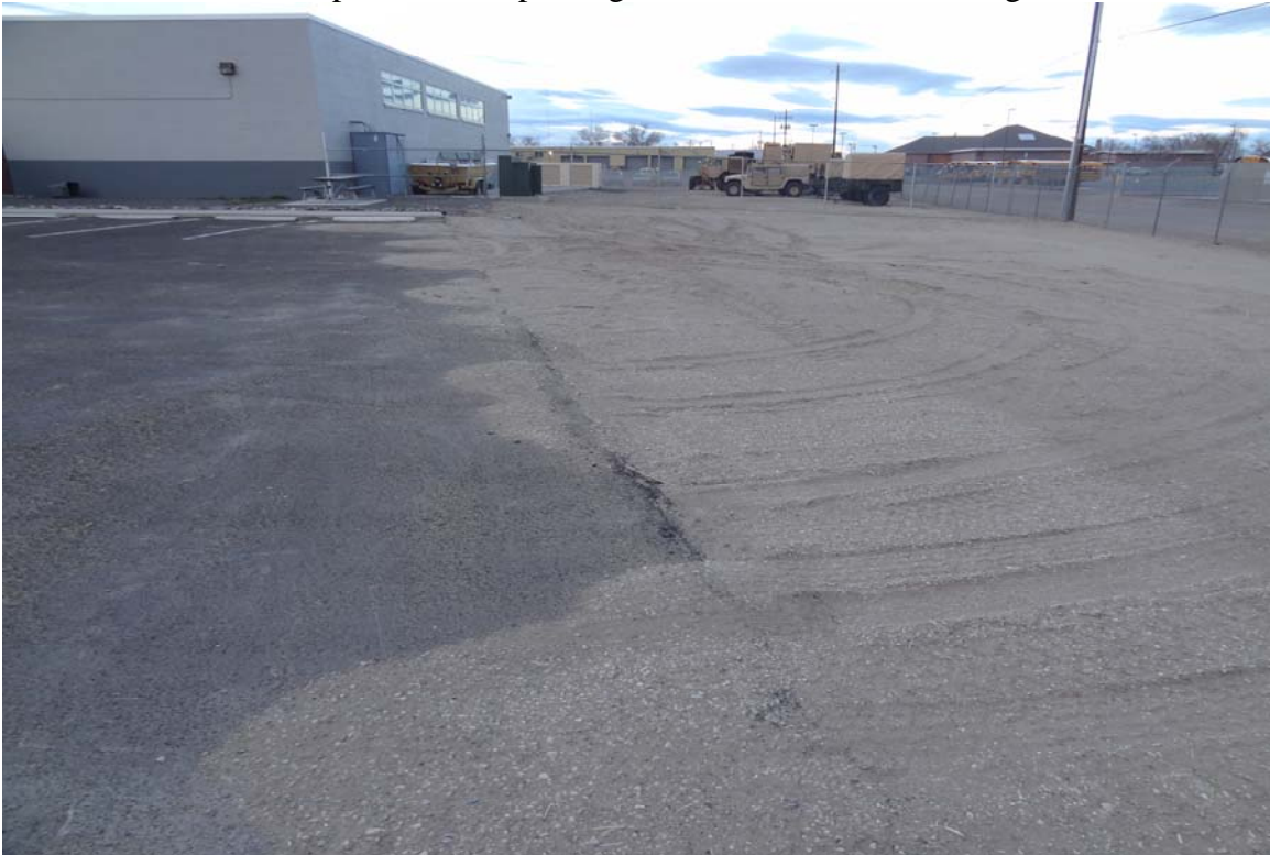
Fallon National Guard Armory Site - Site #9885 Description: Area where paving or soil stabilization is needed.
