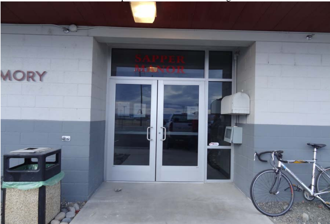
Fallon Armory - Building #0678 Description: Public Entrance.
