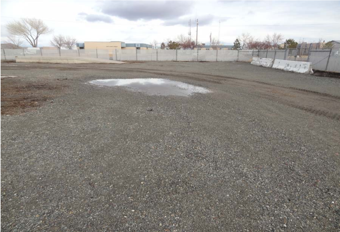
Yerington National Guard Armory Site - Site #9886 Description: Yard area drainage issues.
