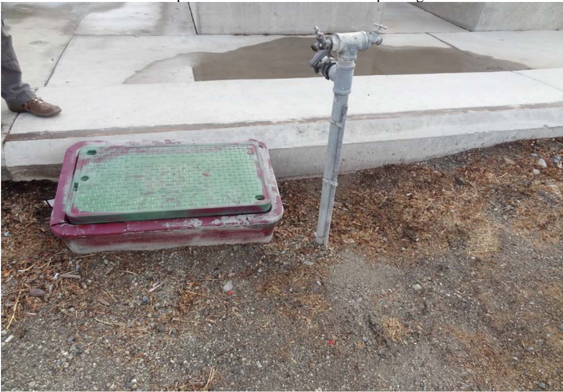
Yerington National Guard Armory Site - Site #9886 Description: Electrical pull box in need of relocation / upgrade.
