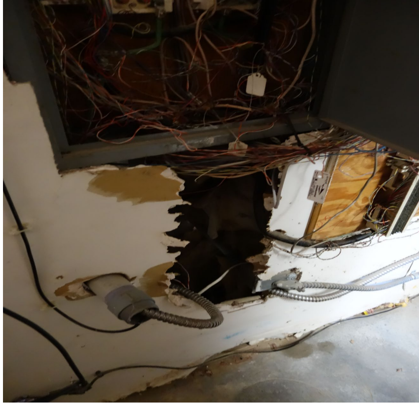
Jean CC NDF Office – FCA Building #2494 Description: Wiring Cleanup & Wall Repair Needed.
