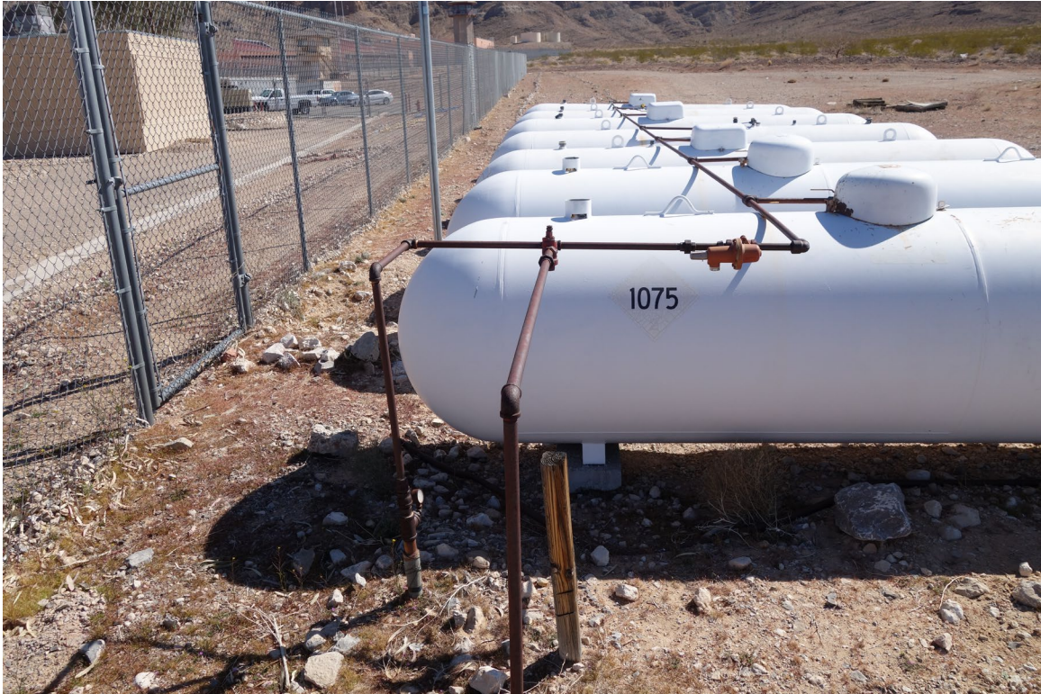
Jean Conservation Camp Site – FCA Site #9892 Description: Seismic Shut-Off Valve for Site Needed.
