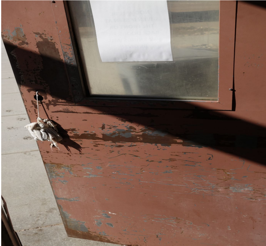
Housing Unit 2 – FCA Building #0662 Description: Exterior Door & Hardware Replacement Needed.
