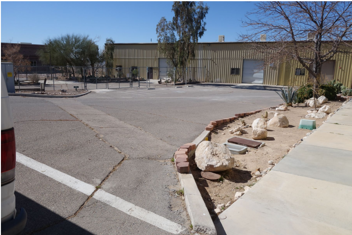
Jean Conservation Camp Site – FCA Site #9892 Description: Crack Patch & Slurry Seal Needed.
