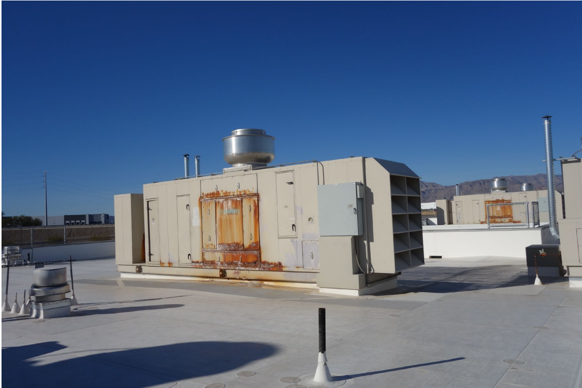
Administration / Housing Units - Building #2457 Description: HVAC Replacement Needed on 2009 Built Housing Units.
