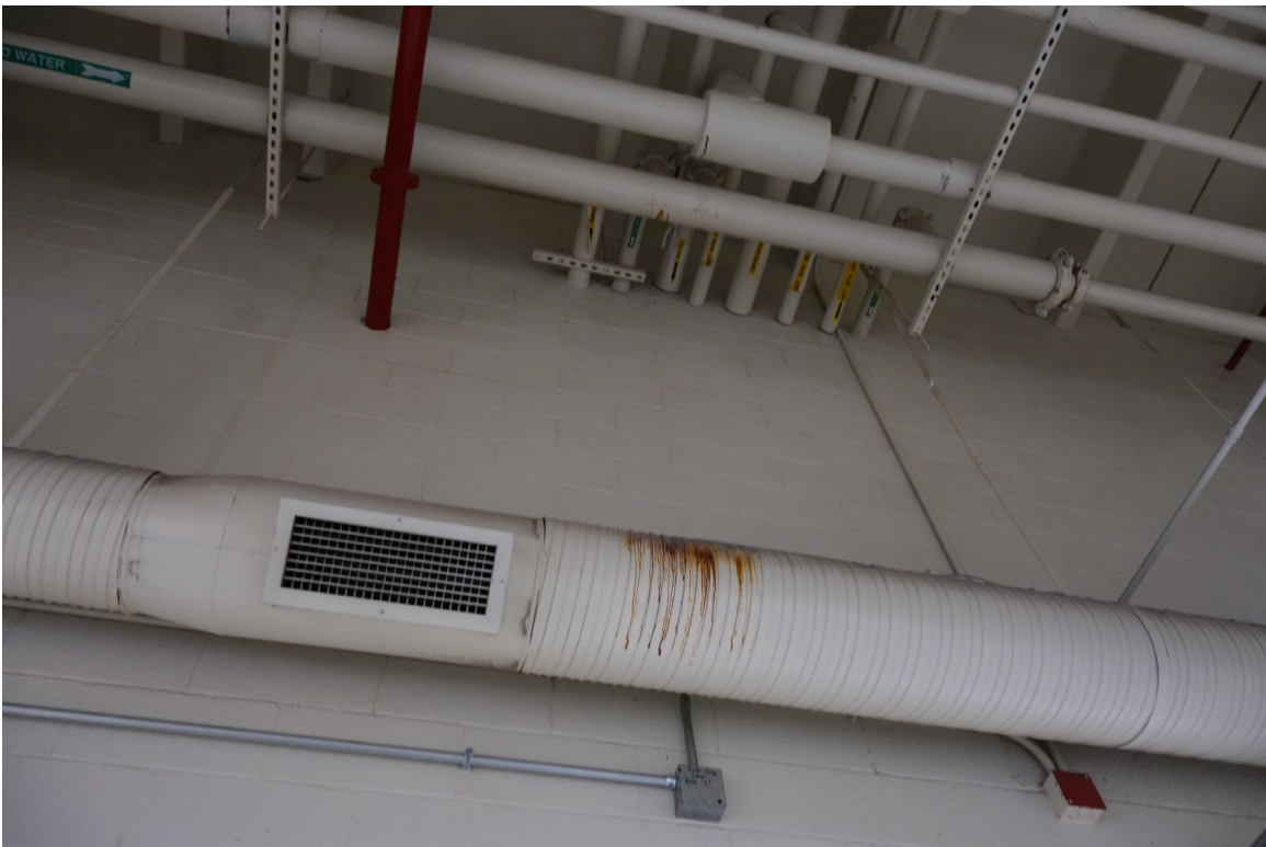
Administration / Housing Units - Building #2457 Description: Domestic Plumbing Replacement Recommended.
