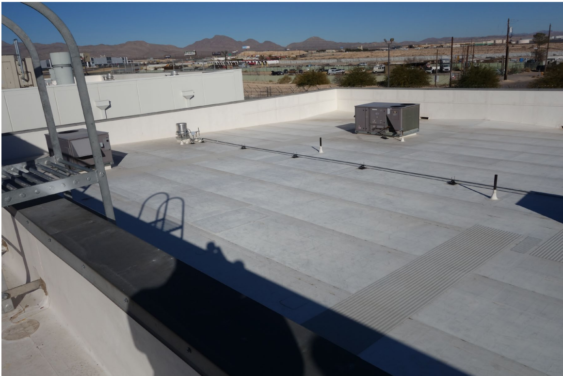
Administration / Housing Units - Building #2457 Description: View of Single Ply Roofing installed in 2014.
