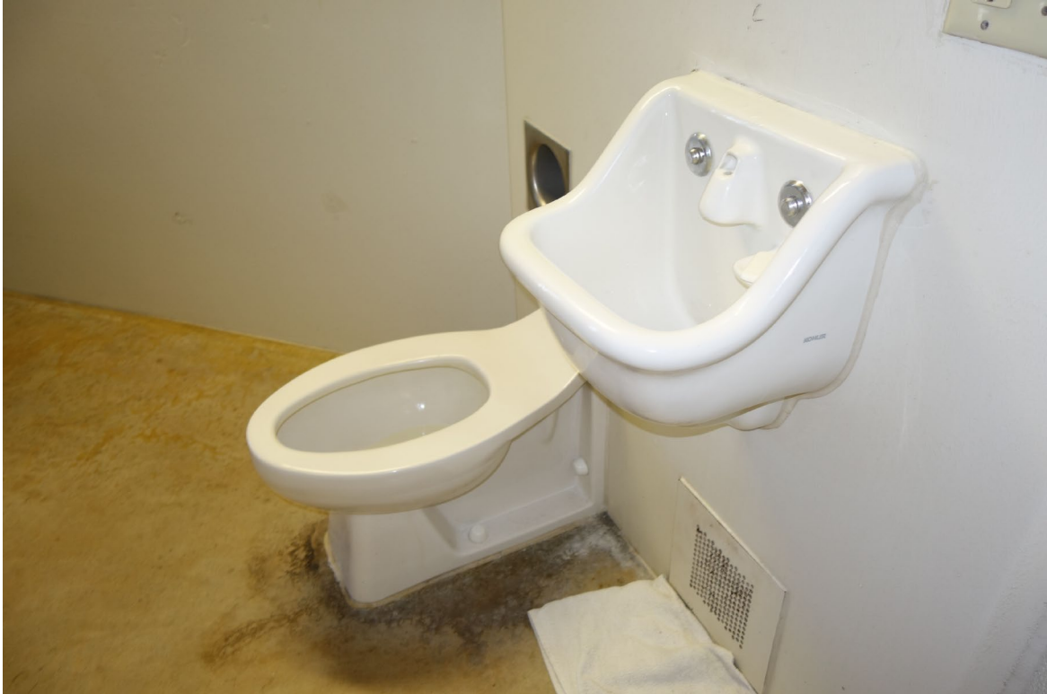
Administration / Housing Units - Building #2457 Description: Plumbing Fixture Replacement to Stainless Steel.
