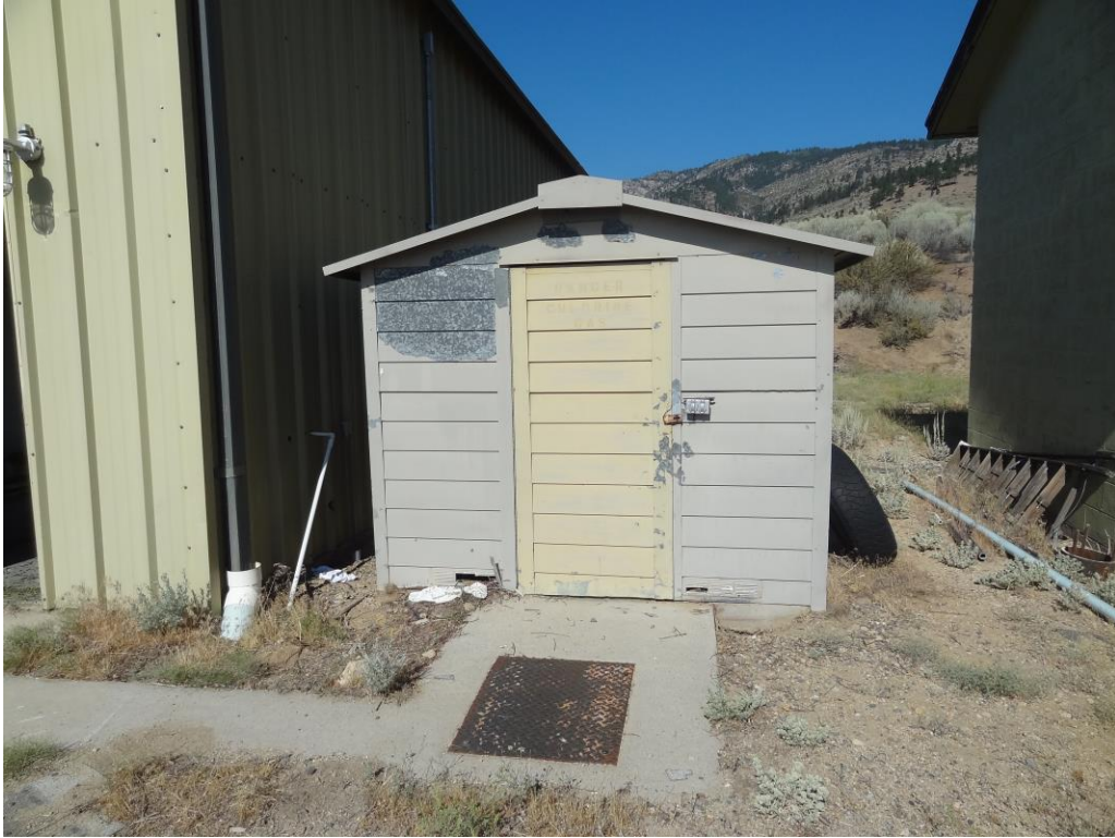
Marlette Lake Storage Shed - Building #2503 Description: Exterior finishes needed.
