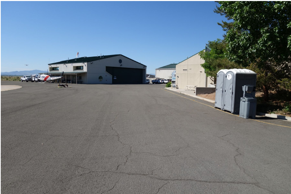
Sierra Front Interagency Hangar – FCA Building #2491 Description: Exterior of the Building.
