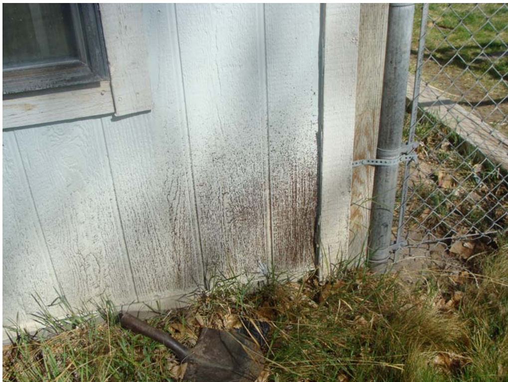
Hatchery Residence 5 - Building #1670 Description: Paint damage from irrigation system.
