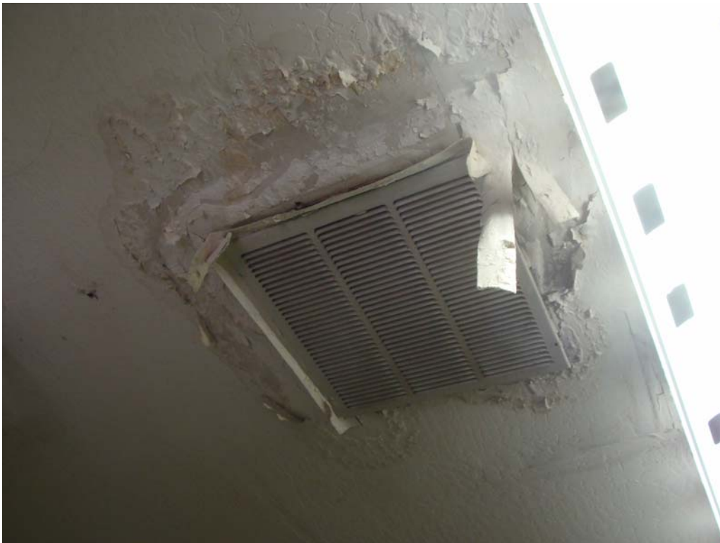
Hatchery Pump House B - Building #1661 Description: Damage to the ceiling.
