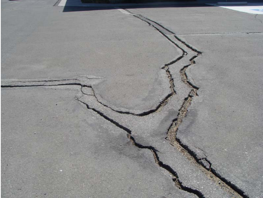
Mason Valley Hatchery - Site #9905 Description: Typical cracks in the pavement.
