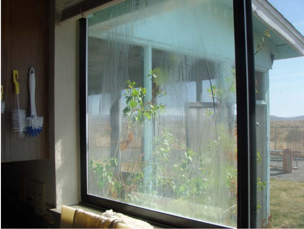
Hatchery Residence 1 - Building #1666 Description: Damaged window seal.
