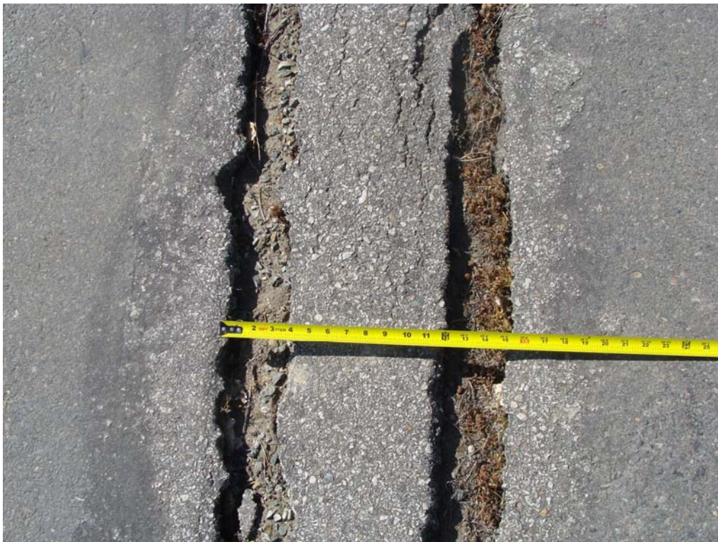
Mason Valley Hatchery - Site #9905 Description: Cracks at east pavement area.
