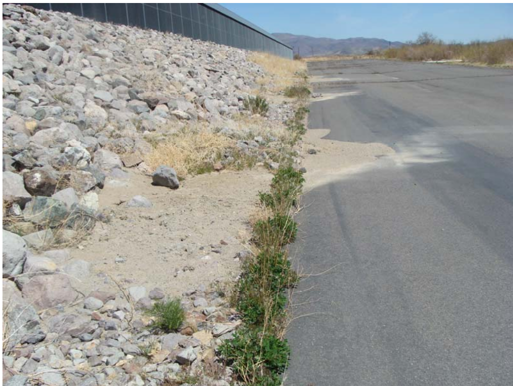
Mason Valley Hatchery - Site #9905 Description: Erosion at rip-rap bank by Raceway.
