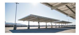
The Solar Carport is a galvanized metal structure supporting photovoltaic panels. The structures are elevated and located over the parking areas to provide covered vehicle parking.
