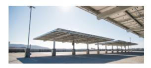
The Solar Carport is a galvanized metal structure supporting photovoltaic panels. The structures are elevated and located over the parking areas to provide covered vehicle parking.
