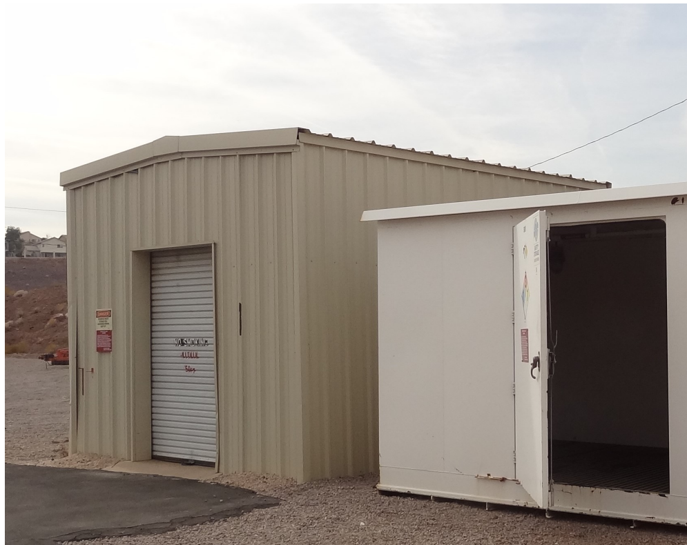
Henderson Armory Hazardous Waste Storage - Building #0684 Description: View of Hazardous Waste Storage Building.
