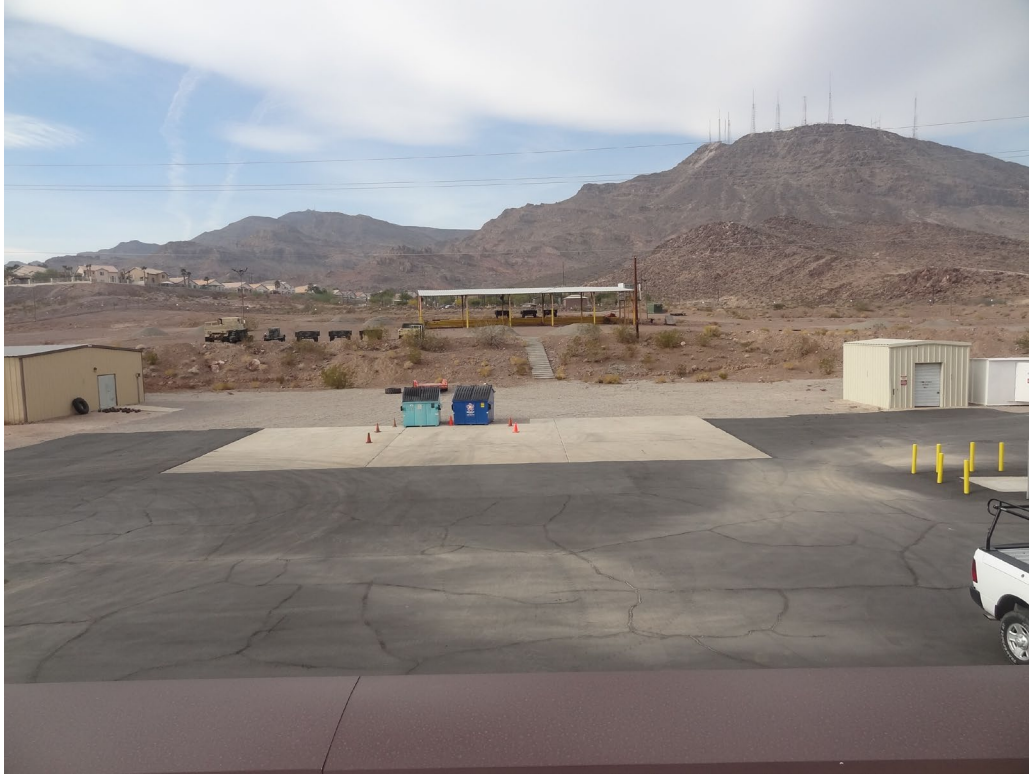
Henderson Armory – Site #9912 Description: Crack Fill & Seal Asphalt Paving.
