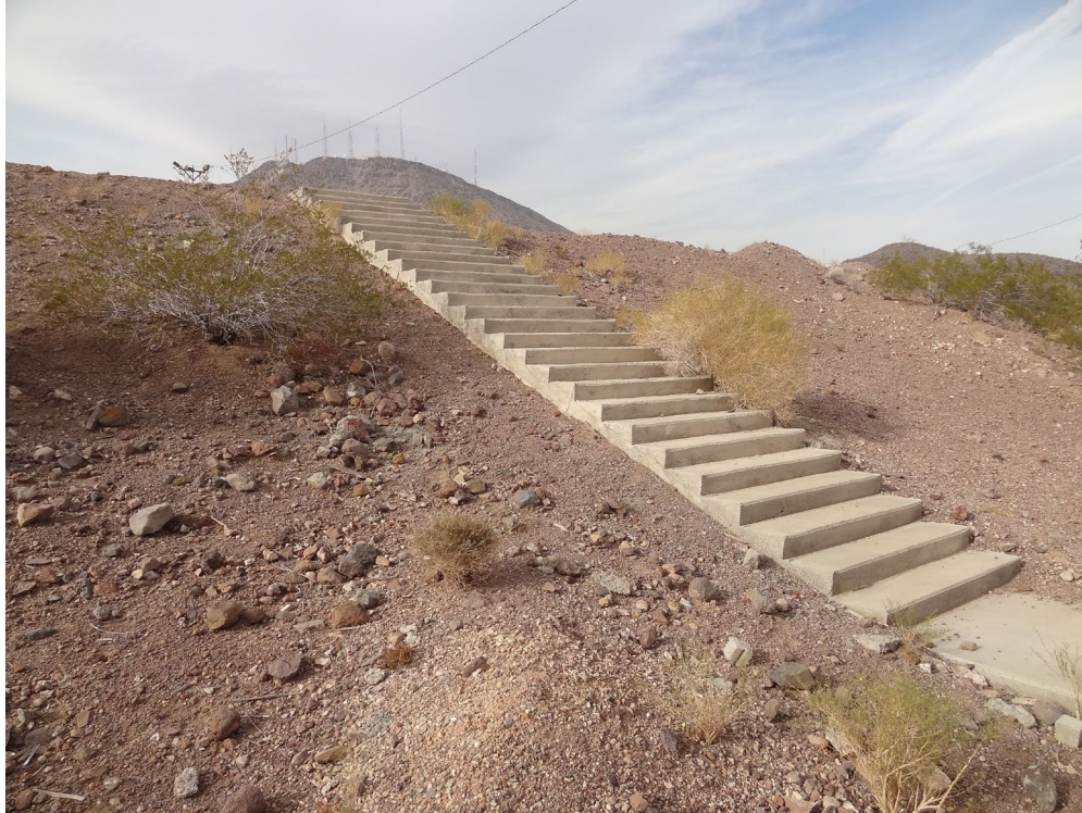
Henderson Armory - Site #9912 Description: Exterior Stair Handrail Installation.
