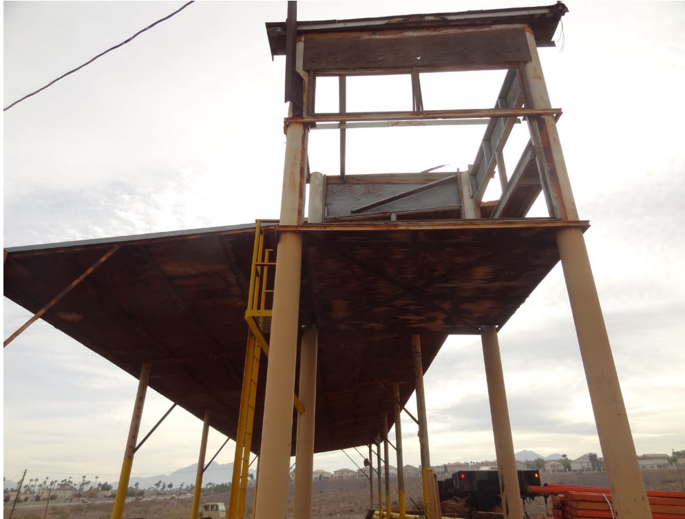
Henderson Armory Range Tower - Building #2412 Description: Guardrail Installation.
