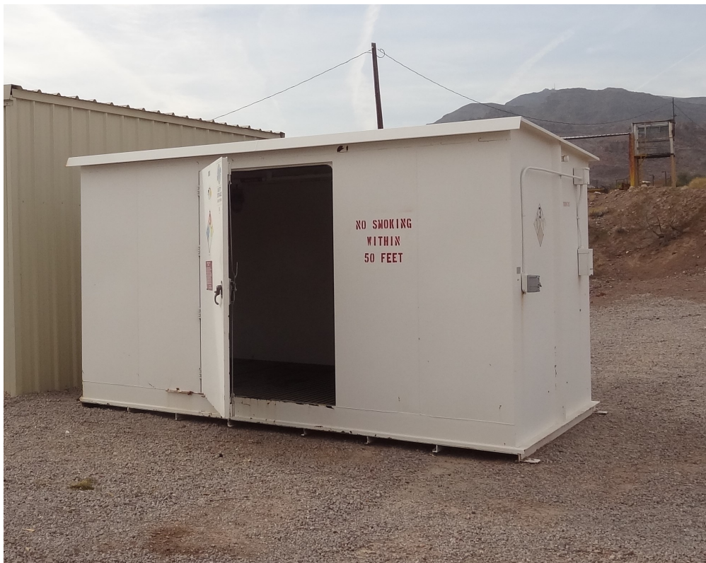
Henderson Armory Oil Storage - Building #3094 Description: View of Oil Storage Building.
