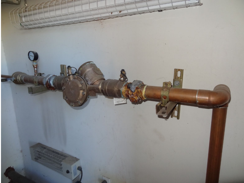
Mormon Fort Visitor's Center - Building #1681 Description: Leaking Back Flow Prevention Assembly.
