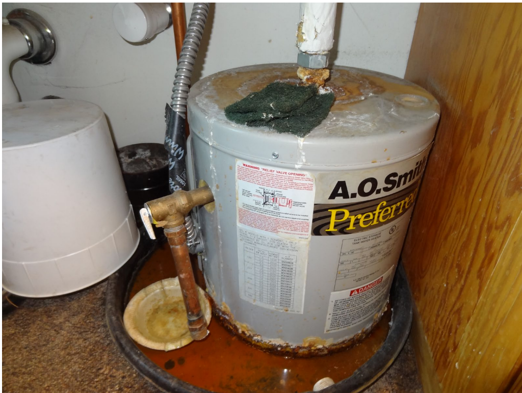
Mormon Fort Visitor's Center - Building #1681 Description: Water Heater Replacement Needed.
