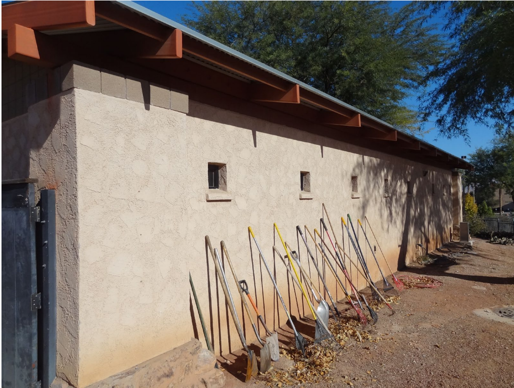
Mormon Fort Vehicle Shop - Building #2397 Description: Exterior of the Building & Need for Drain Gutters.
