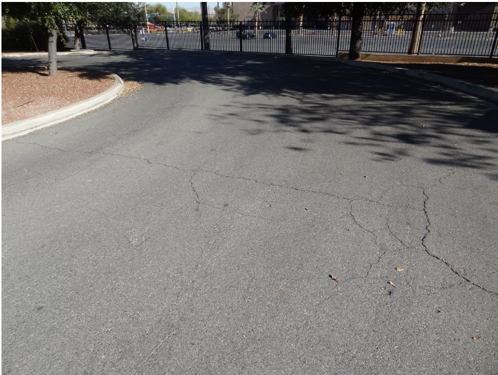
Old Las Vegas Mormon Fort State Historical Park - Site #9913 Description: Crack Fill & Slurry Seal Needed.
