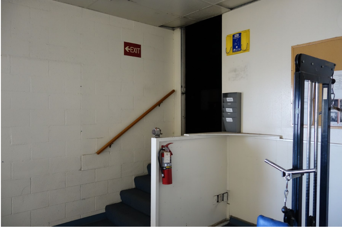
Las Vegas Purchasing Warehouse - Building #2395 Description: Interior Stair Handrail Replacement.
