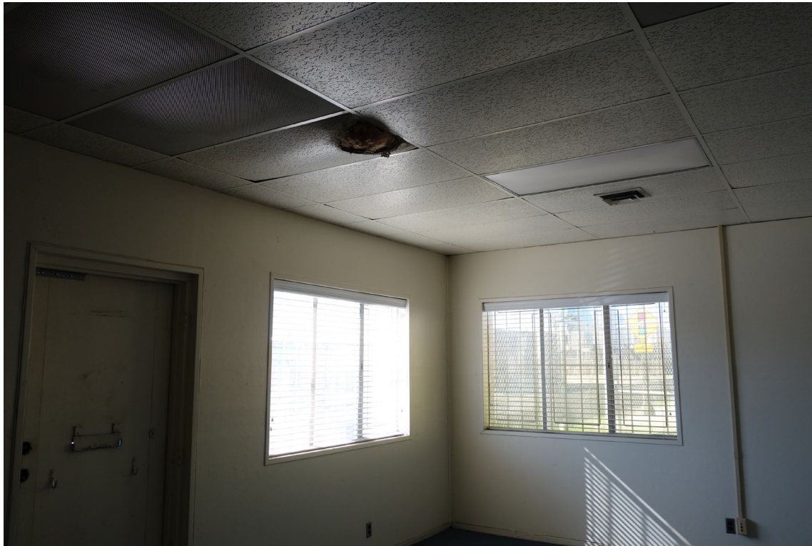
Las Vegas Purchasing Warehouse - Building #2395 Description: Ceiling System Replacement.
