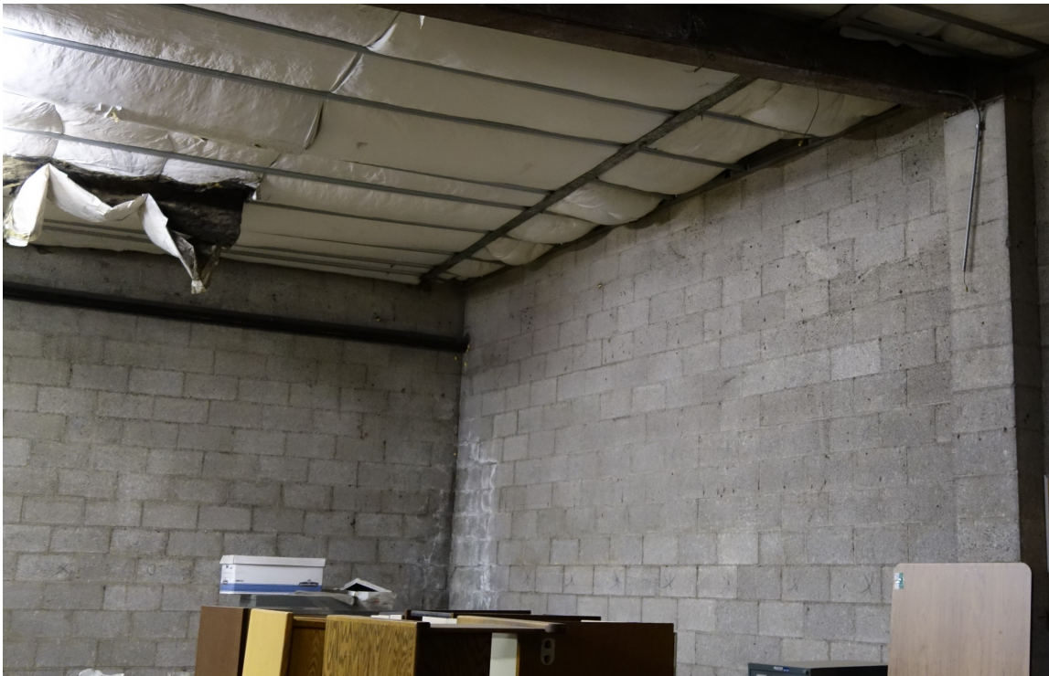
Las Vegas Purchasing Warehouse - Building #2395 Description: Ceiling Insulation Replacement.
