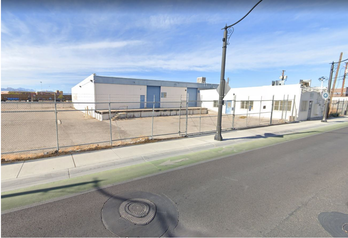
Las Vegas Purchasing Warehouse Site - Site #9914 Description: View of the Site.
