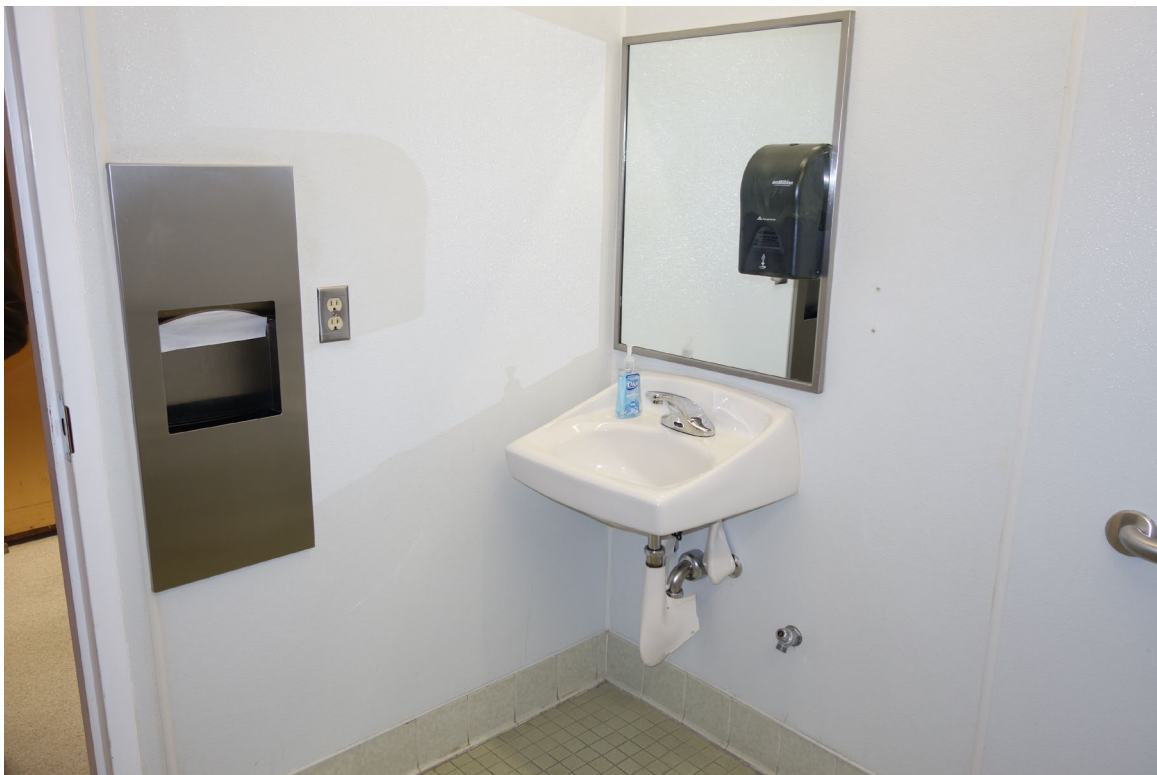
Heroes Memorial Building - Building #0244 Description: GFCI Outlet Installation Needed.
