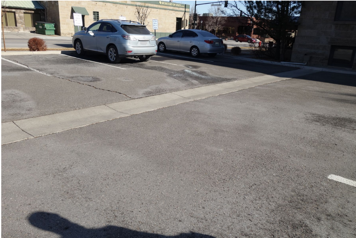
Attorney General Offices Complex - Site #9917 Description: Crack Fill & Seal Parking Recommended.
