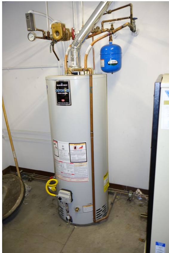
Field Maintenance Shop A - Building #2040 Description: Water Heater Seismic Restraints Needed.
