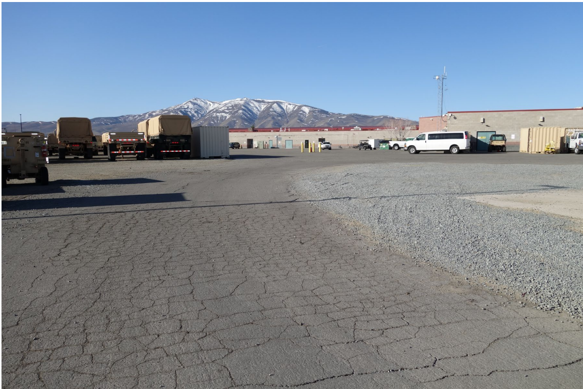
Sen. Harry Reid Readiness & Training Center - Site #9920 Description: Pavement Patch, Crack & Slurry Seal Site Paving Needed.
