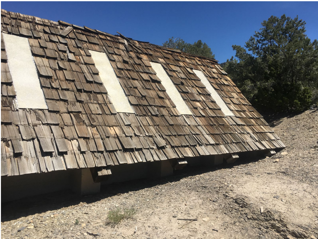
Fossil House Storage - Building #0473 Description: Building Roof Needing Replacement.
