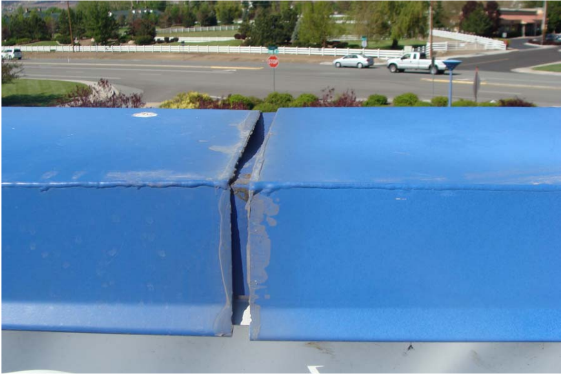
Reno NHP Headquarters - Building #0056 Description: View of cap flashing.
