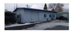
The pre-engineered metal Radio Shop/Dispatch Office includes office, workshop, and storage space. It has two offices, a dispatch wet bar, a unisex restroom, and a non-ADA-compliant ramp. Interior finishes include painted gypsum board, acoustical tile ceiling, and carpet. Climate control is provided by a gas-fired FAU with an exterior condenser, Smoke detection is installed.
