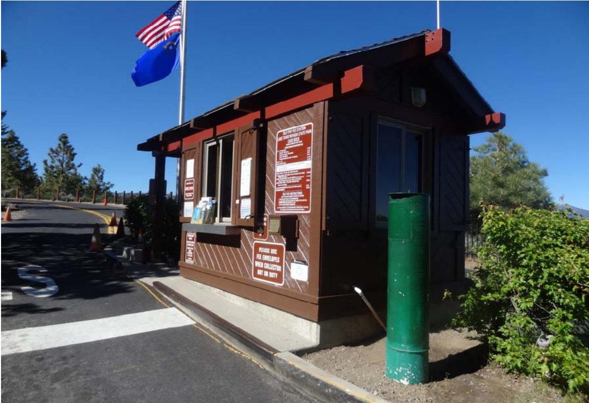
Cave Rock Fee Station – FCA Building #0588 Description: Exterior of the building.
