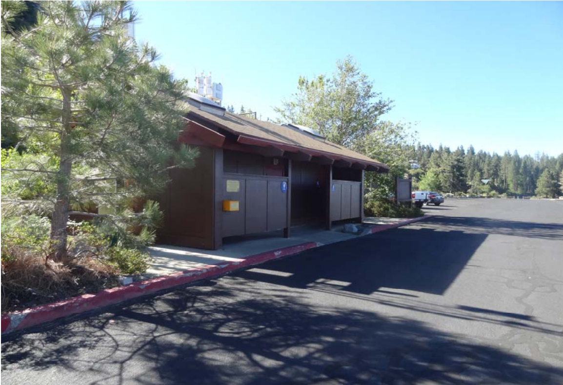
Cave Rock Comfort Station – FCA Building #0597 Description: Exterior of the building.
