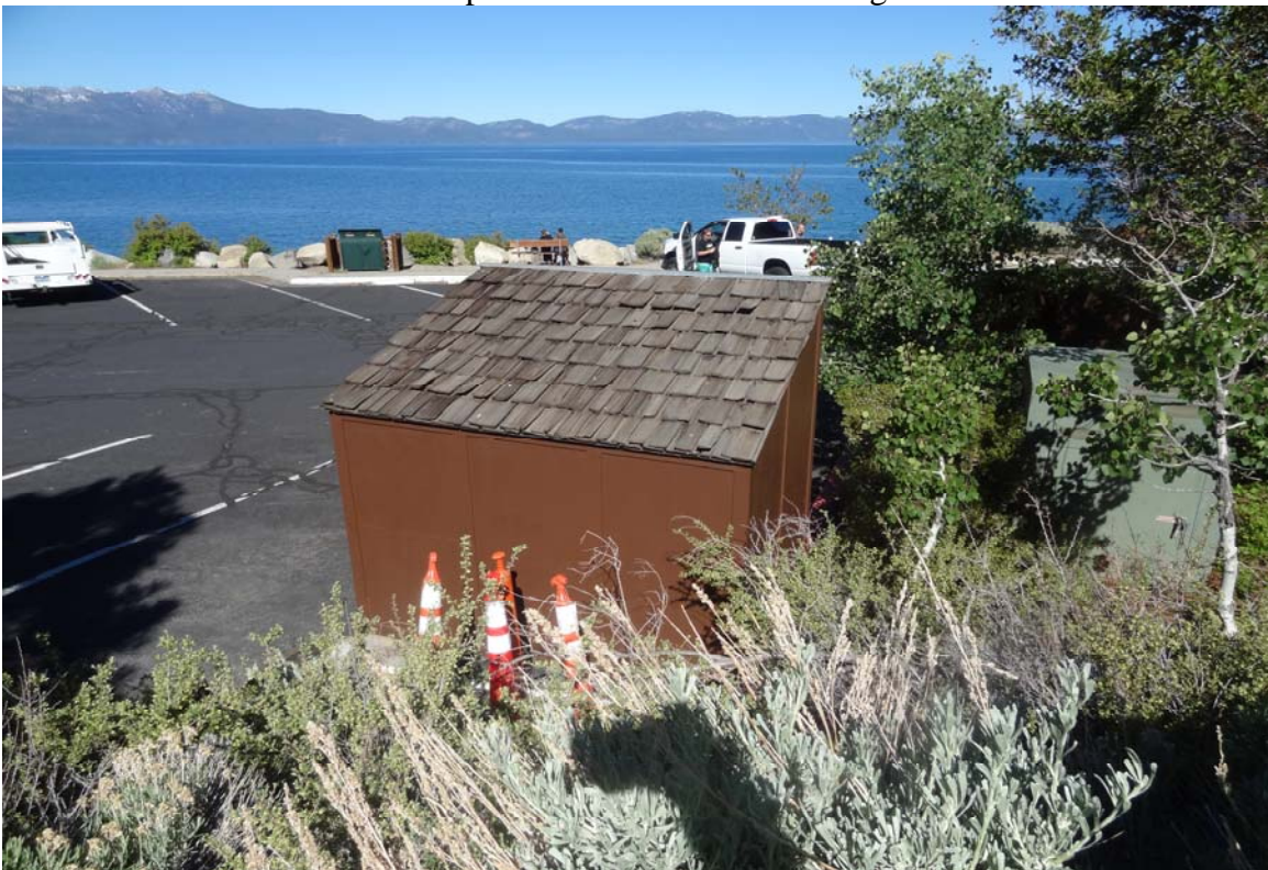
Cave Rock Storage Shed – FCA Building #0586 Description: Exterior of the building.
