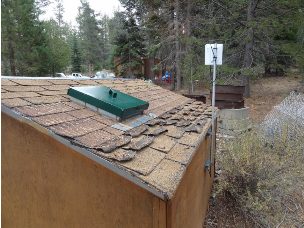
Pump House – FCA Building #1325 Description: Roof in need of replacement.
